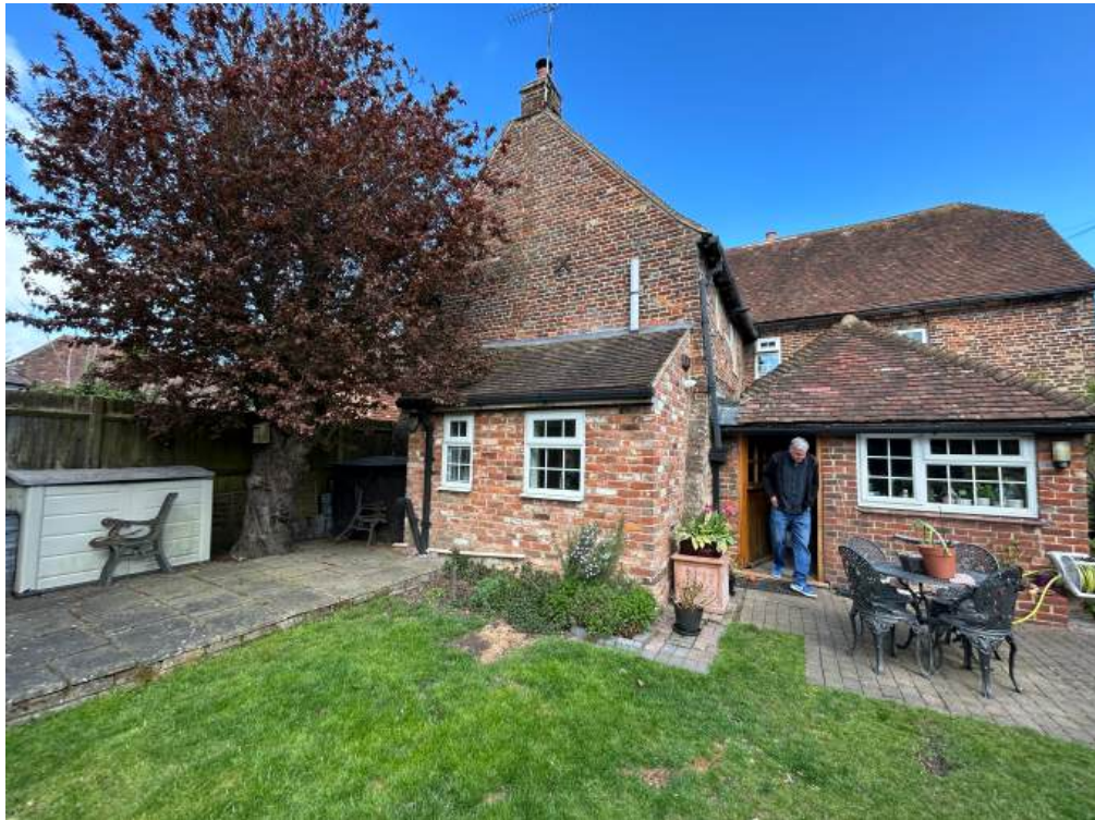
View of rear elevation from the garden.
