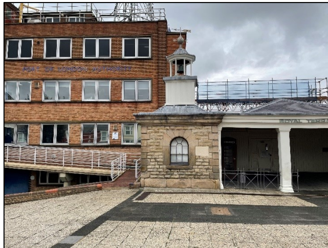
Figure 4: View of western pavilion of RTP with the link behind
