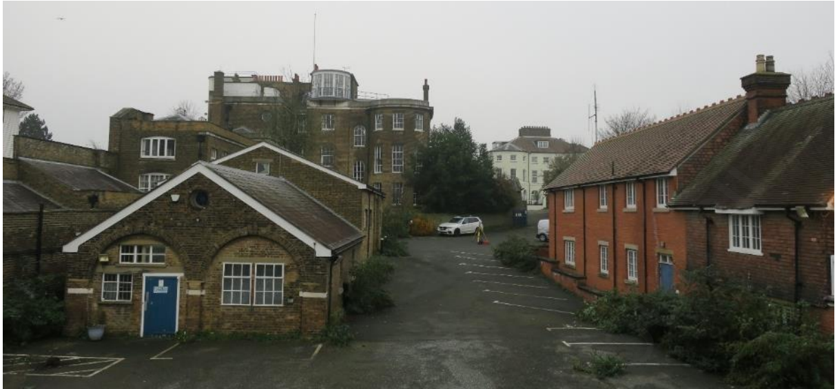
Fig 29 View from the flood wall to the north, showing the rear elevation with boathouse and former coastguard station in front and in the background Whitehall Place while on the far left the corner of the Heritage Quay development
