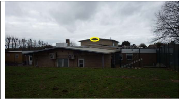
Plate 13: Recommended area on school building for bat box.
