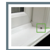
Drainage Channel
