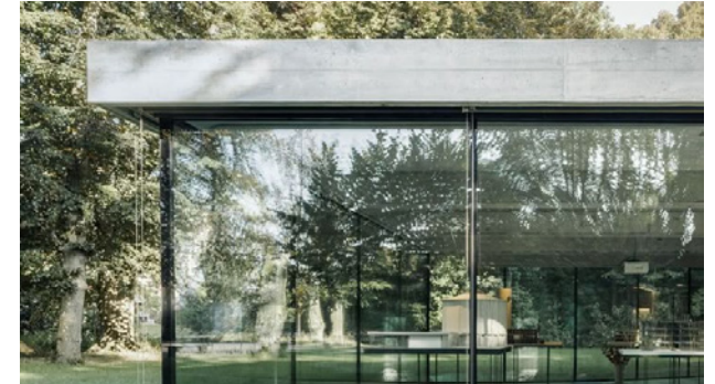
Flat roof form
