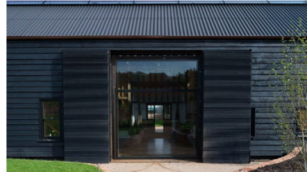
Large openings and expanses of glass
