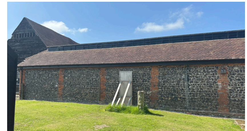
6 Building 14, Whitehouse Farm
