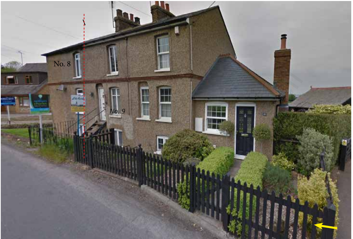
Heading into village along Forge lane looking to row of terraces to right
