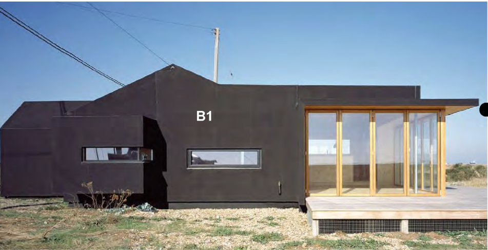
Black Rubber House in Dungeness by Simon Conder Associates.
