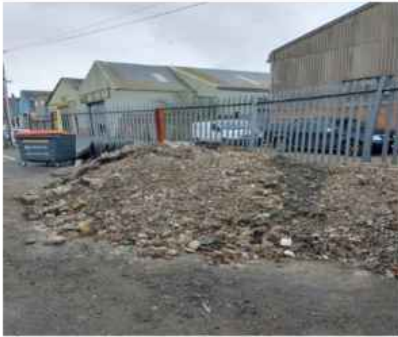
Figure 5: Stockpile of general building material comprising concrete, tarmac, stone and gravel located on the northern boundary close to the site entrance.
