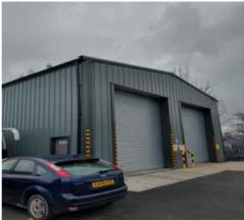
Figure 7: Looking south-east – main structure on site currently in use as the coach servicing building. Note the palisade fencing to the R.H.S of photo frame marks the southern boundary.
