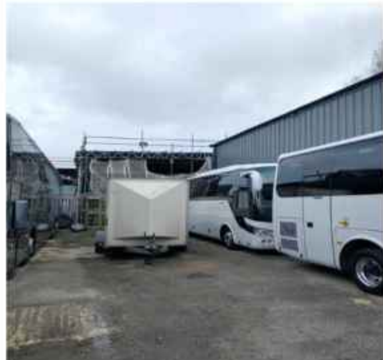
Figure 8: Looking east - Lay down area for the coaches. Note the existing Coach servicing building to R.H.S of photo frame. The proposed development is an extension of the existing structure which will cover most of the area in the photo. Note concrete hardstanding throughout the east of the site.
