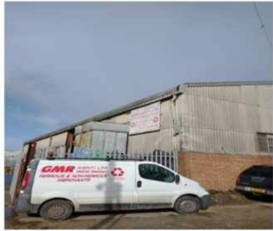
Figure 2: Looking north – Metal works situated directly opposite the site (approx. 10 m from site entrance).
