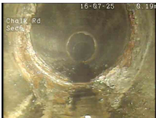
SW1AX_9eb4e2d5-8a46-406b-bfb7-429fa7d84ddd_20250725_132735_570.jpg, 00:00:09, 0.50 m Attached deposits, encrustation at joint from 2 o'clock to 10
