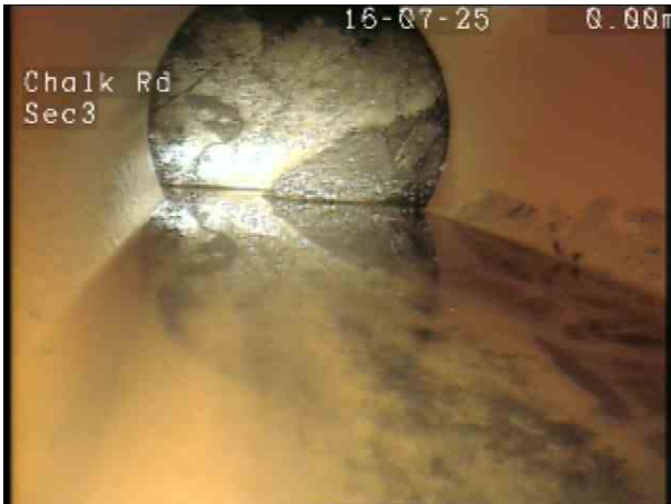
SW3X_bf7640f8-40f4-46dc-b646-70954f421e66_20250725_130109_255.jpg, 00:00:02, 0.00 m Water level, 10% of the vertical dimension
