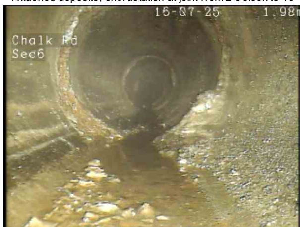
SW1AX_fdb3f9d8-27bb-48f3-9dce-ada41a5fc1a5_20250725_132823_531.jpg, 00:00:31, 2.40 m Attached deposits, encrustation at joint from 3 o'clock to 10
