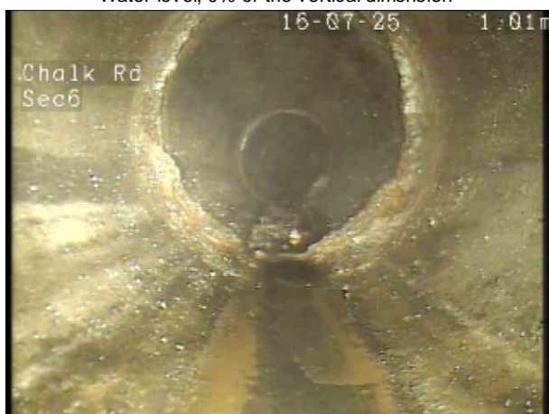
SW1AX_f4cfc597-a243-4a1d-af56-ecb7cdf0f259_20250725_132758_269.jpg, 00:00:19, 1.40 m Attached deposits, encrustation at joint from 12 o'clock to 12
