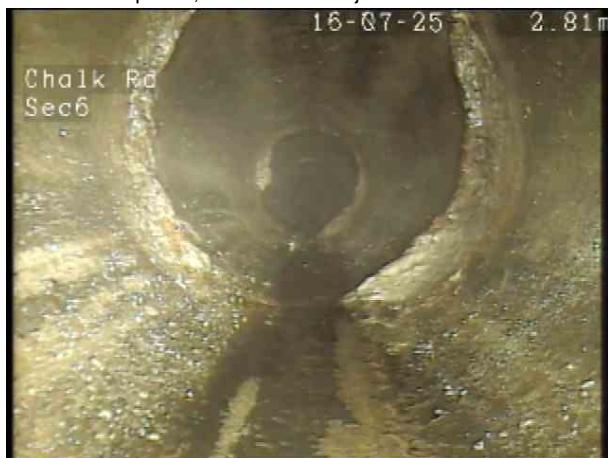
SW1AX_c73c694e-add2-4a94-8c46-028ac5980726_20250725_132846_514.jpg, 00:00:44, 3.10 m Attached deposits, encrustation at joint from 12 o'clock to 12
