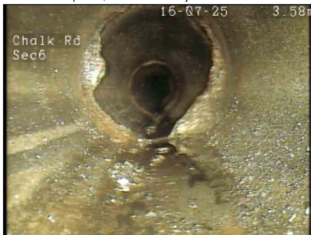
SW1AX_9fc44344-6ee2-4eb1-99c6-bb8b1bb80b1f_20250725_132908_245.jpg, 00:00:54, 4.00 m Attached deposits, encrustation at joint from 12 o'clock to 12
