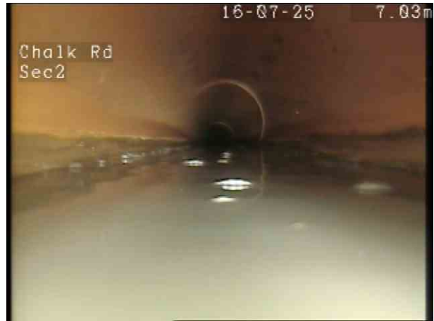
SW2X_06134f88-0cfb-48ce-86b8-16c43289cae0_20250725_125627_995.jpg, 00:01:30, 7.00 m Water level, 25% of the vertical dimension
