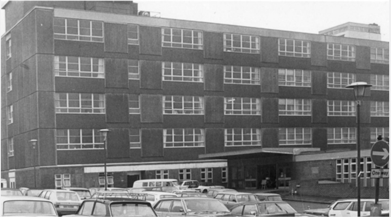
Gravesend Hospital Block M in its original form. The building was completed in 1971.
