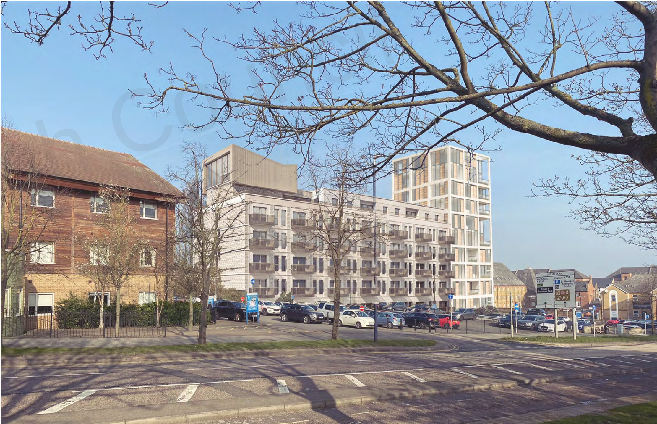
Gravesend Hospital Block M
