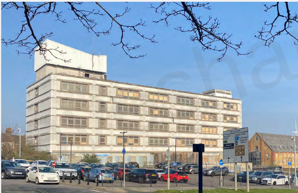
Gravesend Hospital Block M
