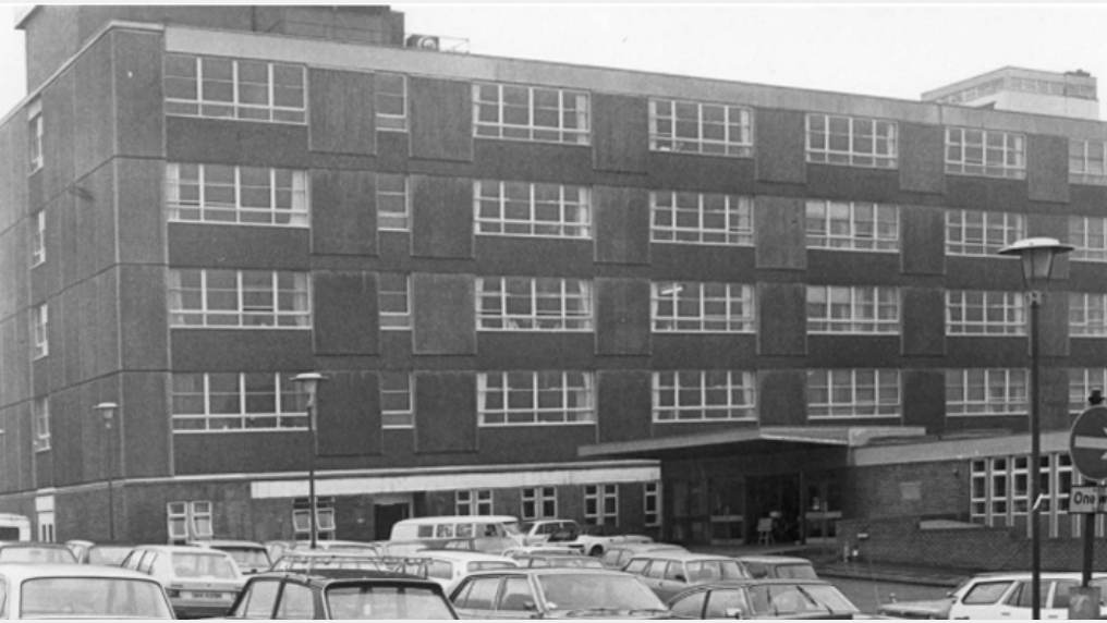
Gravesend Hospital Block M
