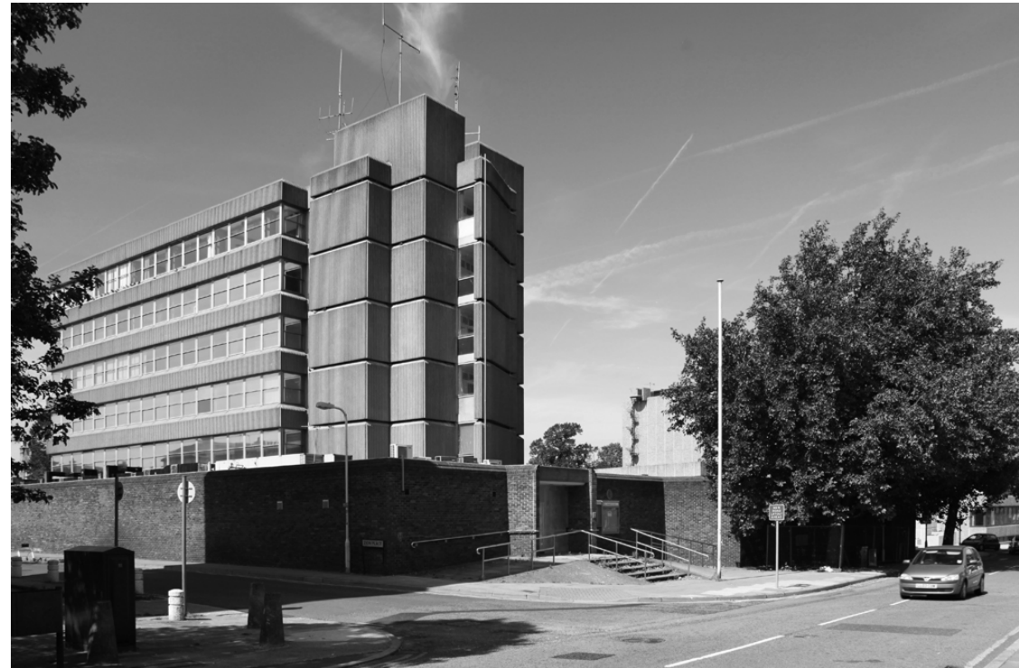
View looking north down Windmill Street
