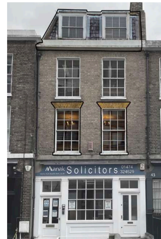
Splayed brick header in contrasting brick with dormer windows to slate roof.
