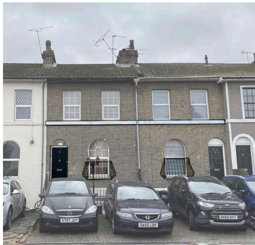
Georgian proportion windows with juliette balcony and splayed window header. Decorative render banding contrasting with brick.
