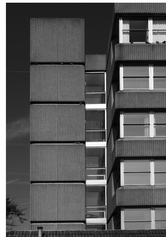
Detail bay of concrete facade
