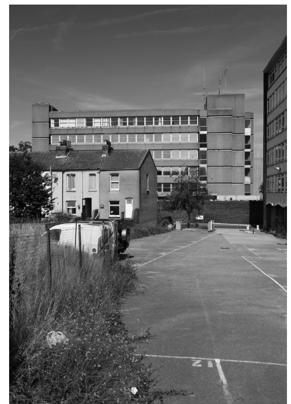
View from rear of Cygnet House looking North
