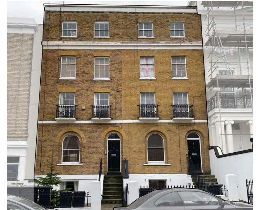
Five-storey terrace pair with contrasting buff brick. Decorative banding, splayed window headers, Juliette balcony, clear hierarchy of window proportions.
