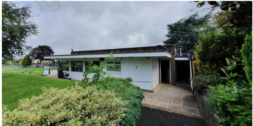
Fig 14—View of Pro shop and entrance to Trolley/ Buggy store
