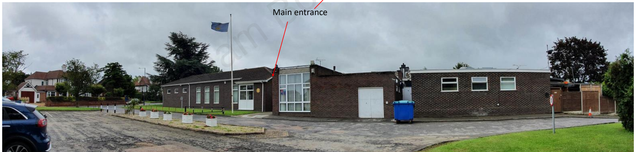
Fig 9—Front view of Clubhouse
