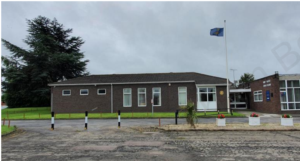
Fig 13—Front view showing added pitched roof to Admin area
