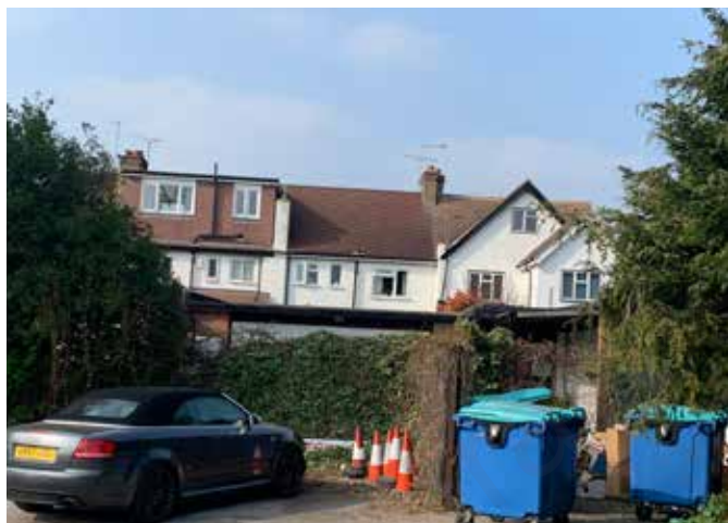
Close Neighbours A: Dennis Road South. Some of the upper windows of these houses directly overlook the Golf Club car park and Club House.
