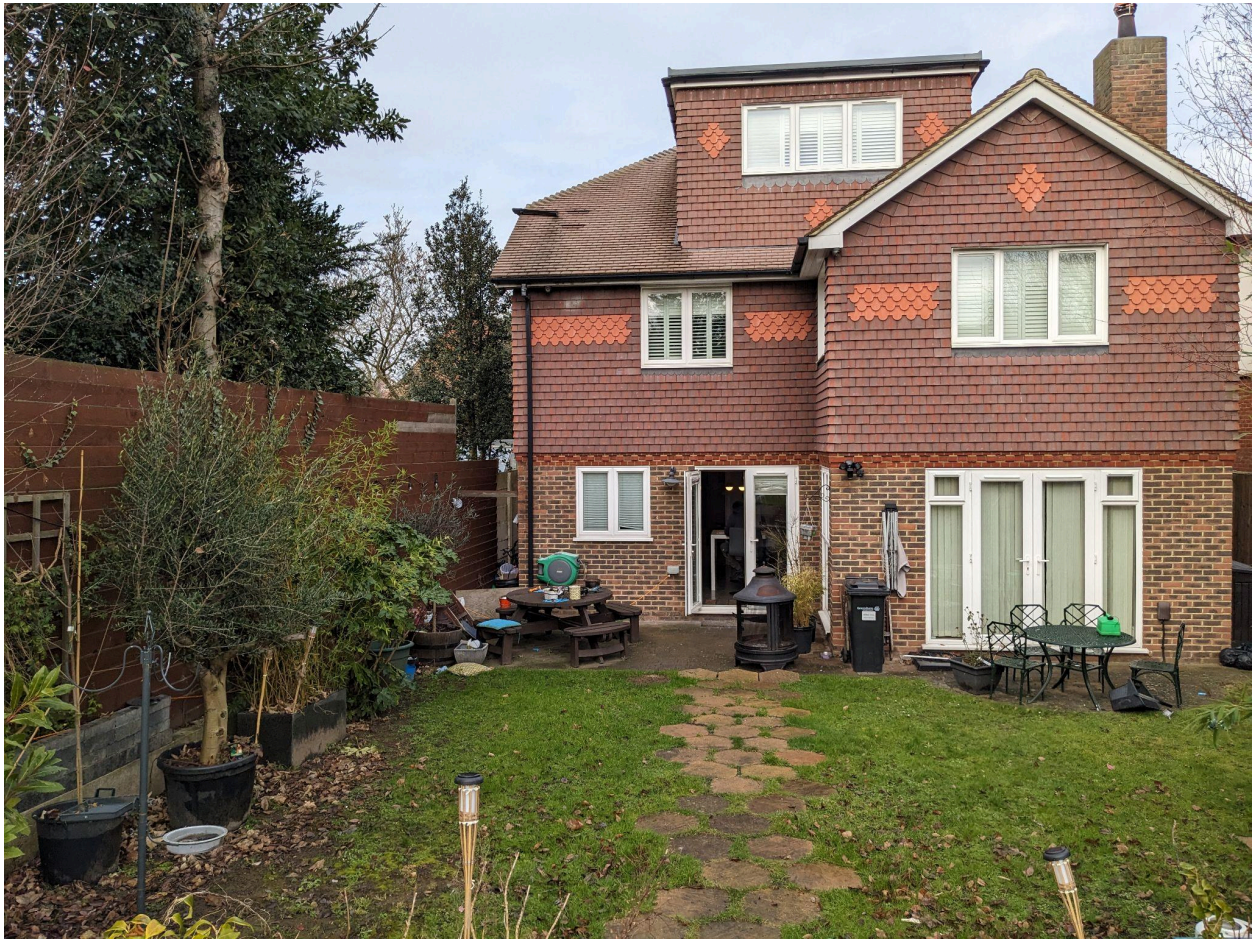
Existing rear elevation of the property, with dormer extension
