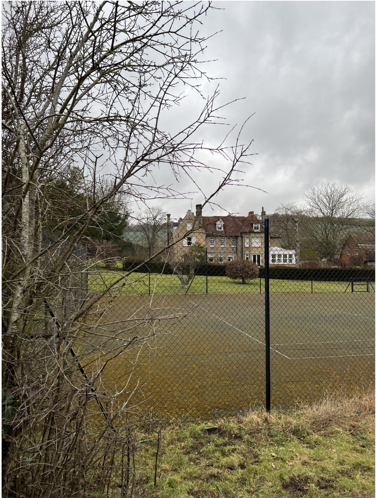
Rear elevation of the dwellinghouse seen from within the application site behind the tennis courts.
