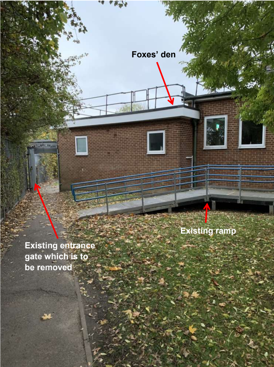
Existing narrow gate, pathway and ramp
