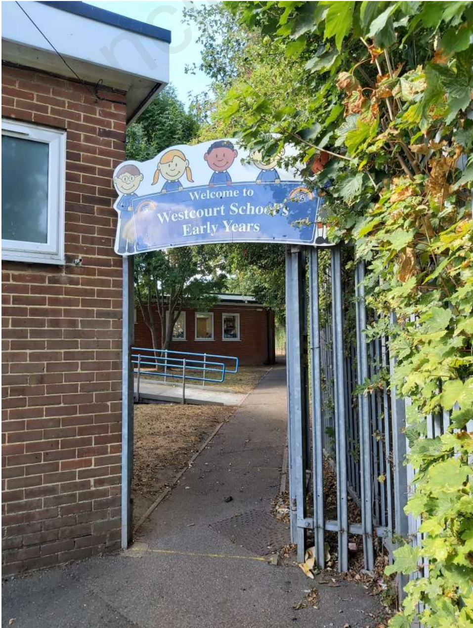
Existing narrow gate and pathway to nursery, reception and breakfast club which is to be removed
