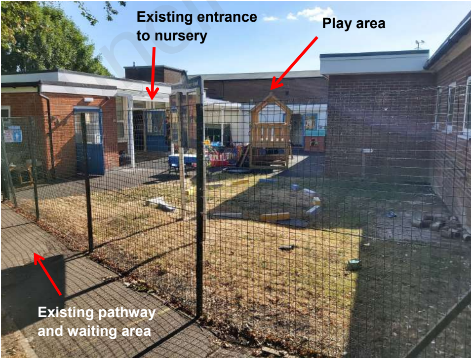
Existing entrance to the nursery and curved waiting area
