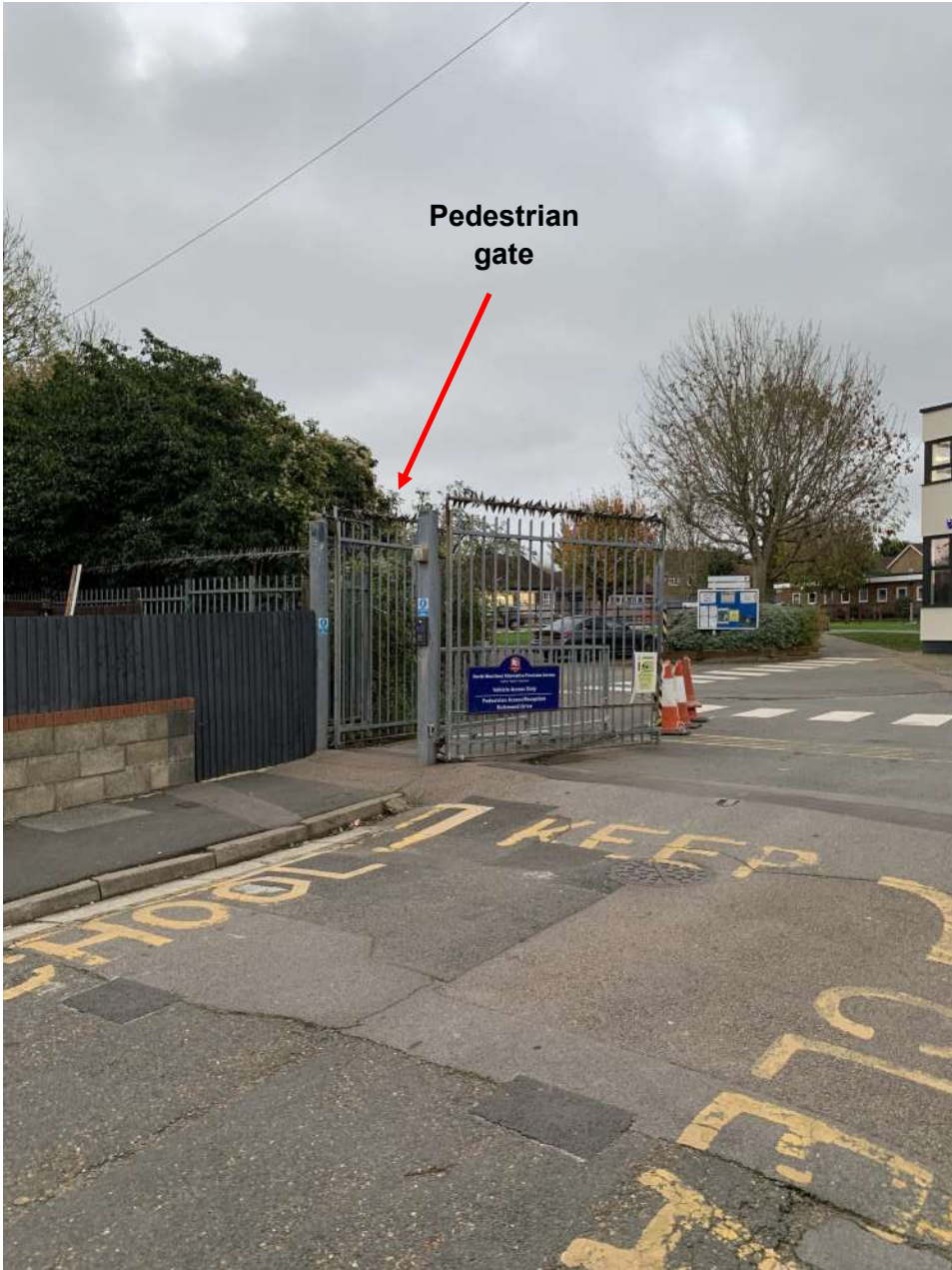
View of the pedestrian gate sited to the left hand side of the vehicular entrance gate
