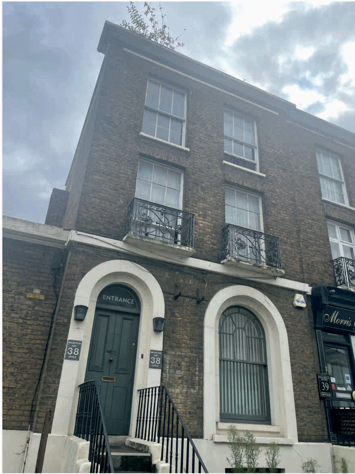
EXTERIOR - Front elevation with entrance facing Windmill Street
