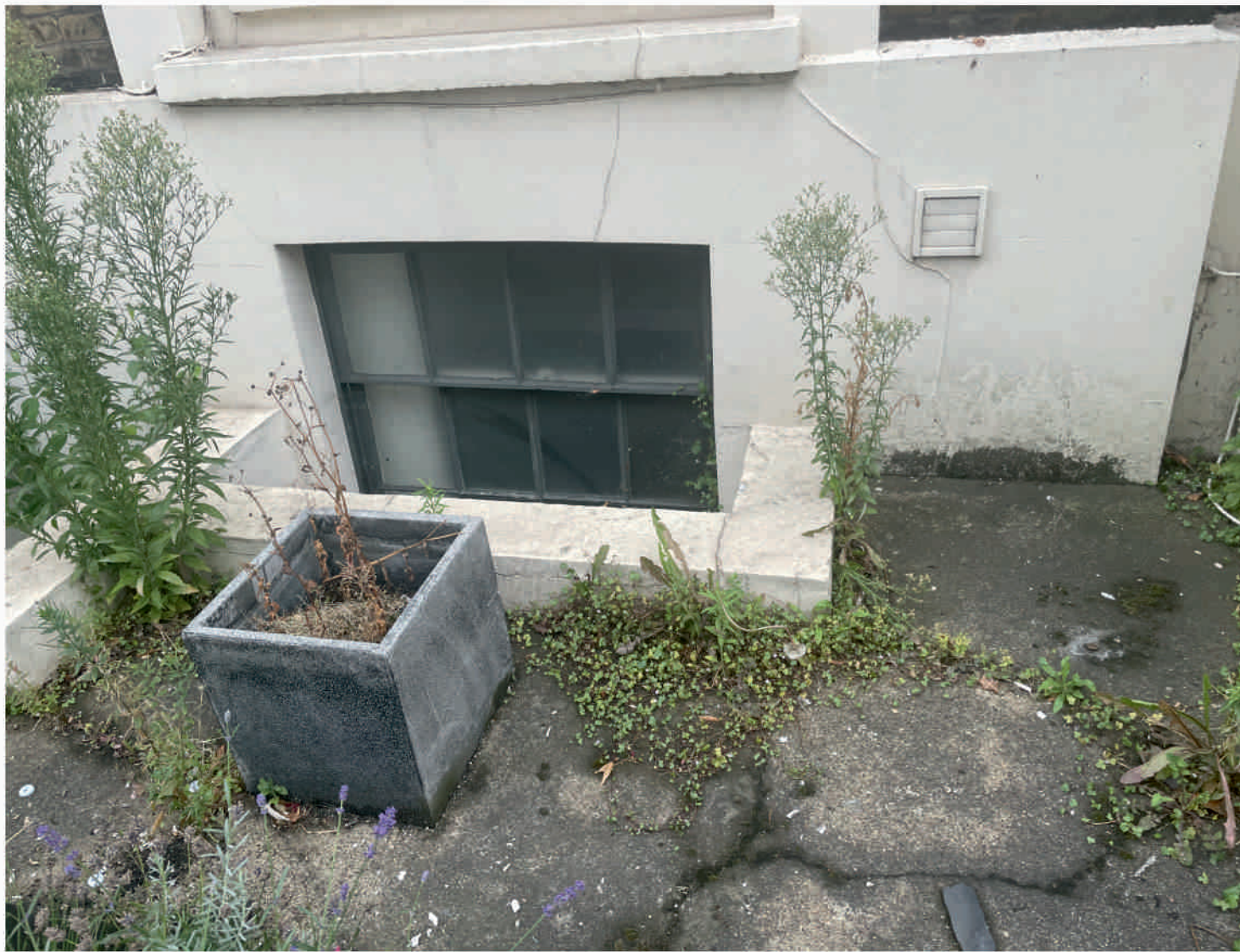
EXTERIOR - Light well and basement window
