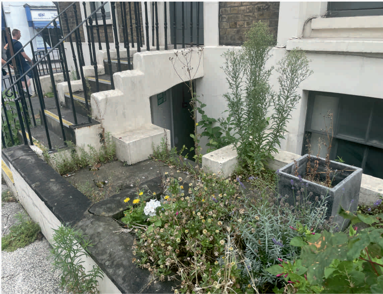
EXTERIOR - Under access stair entrance to basement
