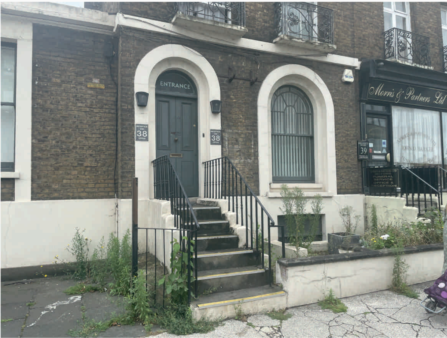
EXTERIOR - Front view from footway of Windmill Street showing basement window, light well and entrance steps
