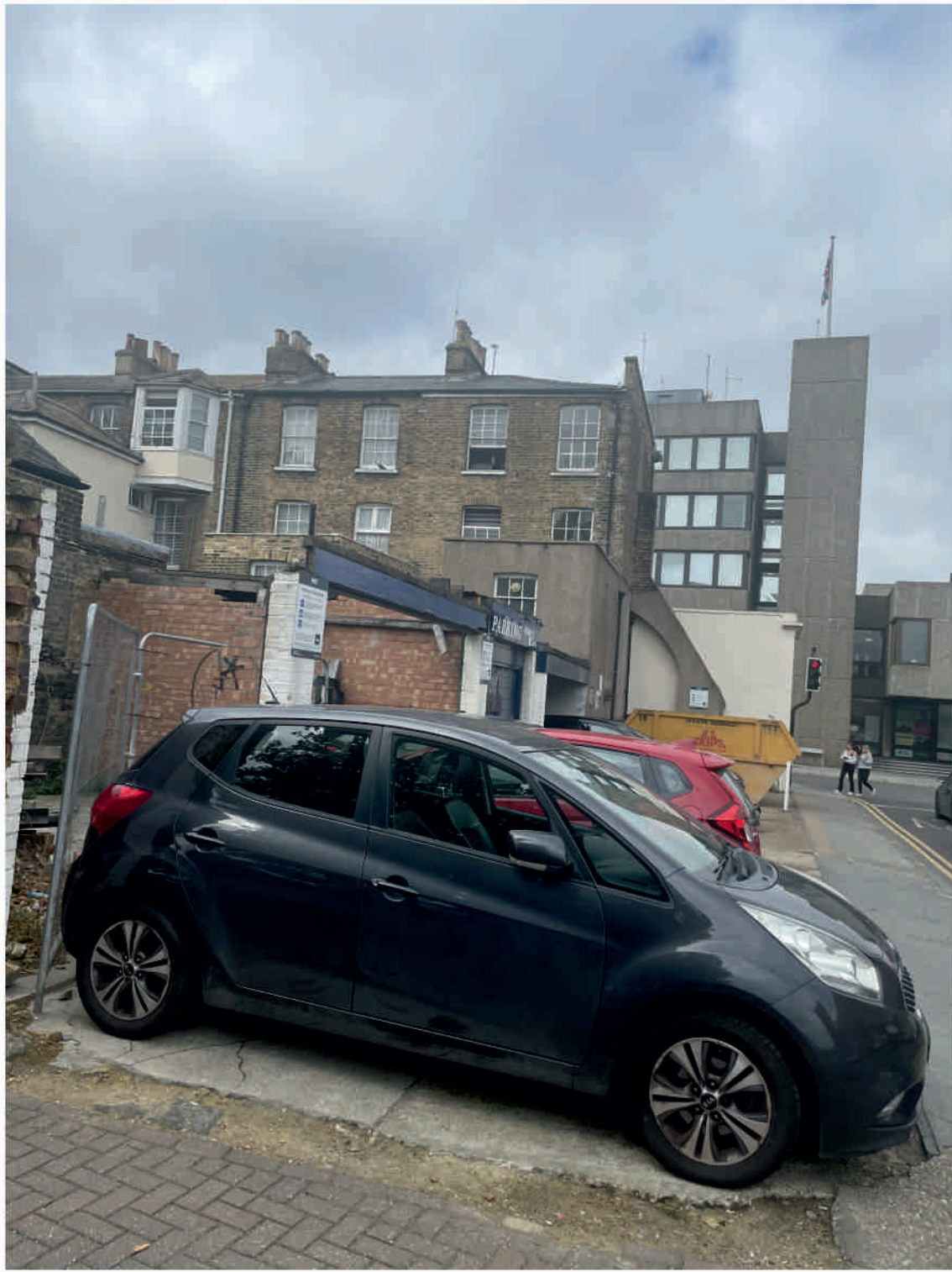
EXTERIOR - Rear of building showing part demolished garages and existing parking forecourt on to Lord Street
