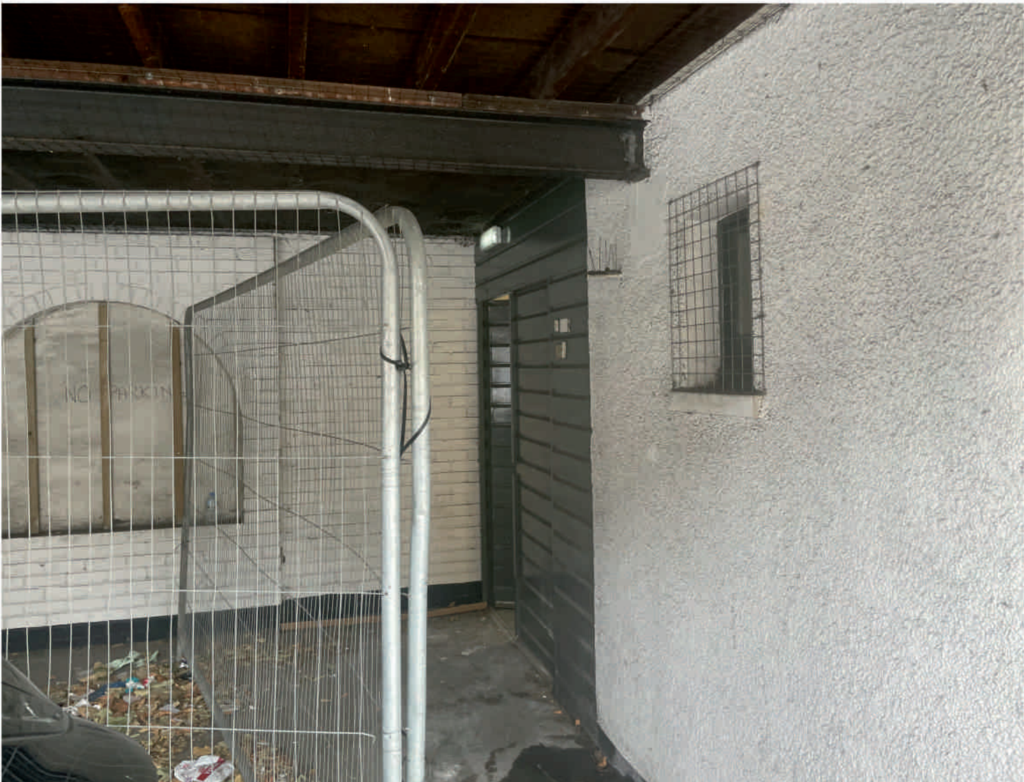
EXTERIOR - Rear doors at rear under car port
