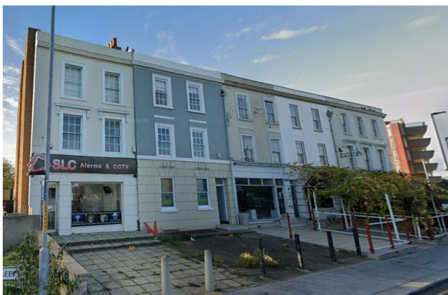
View of 20-24 Stone Street from south-west on corner of Stone Street and Rathbone Road
