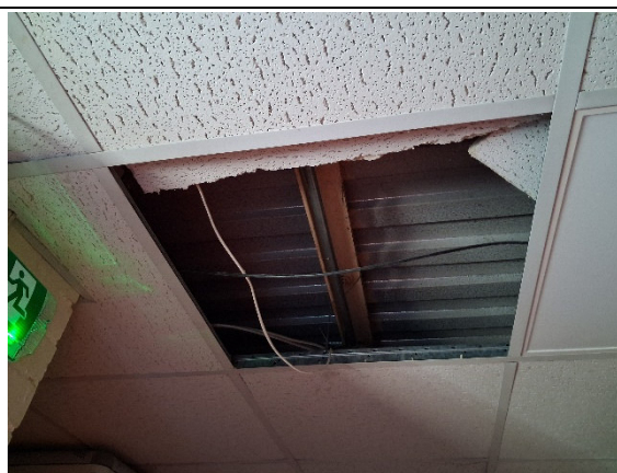
Plate 16. False ceiling leading to cavity from inside building.
