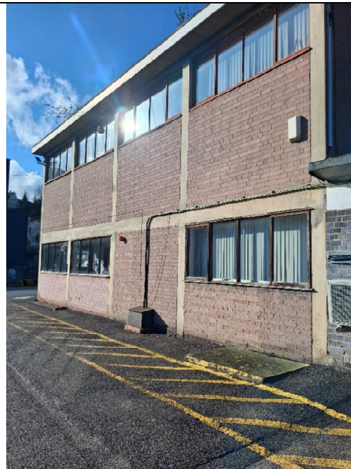
Plate 14. Exterior of building proposed for removal.
