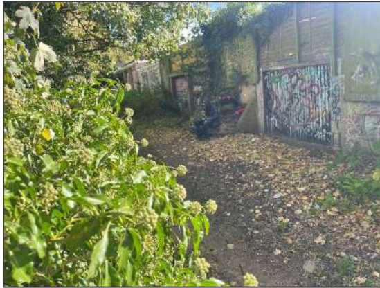
Photograph 4.2 - Wall at the north boundary of properties along Parrock Avenue
