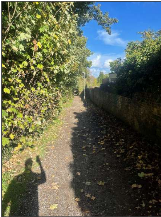
Photograph 4.2 - Wall at the east boundary of properties along Milton Hall Road
