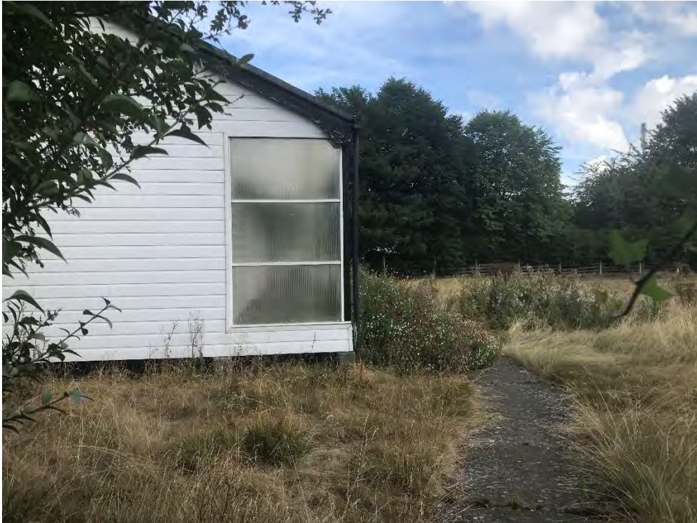
Figure 11 View of the Pavilion as seen from the south
