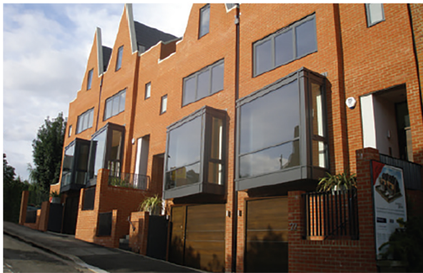
[2] Windows* & External Doors UPVC windows + Comar 7 doors (RAL 7016 - Anthracite Grey) * including patio / french doors
