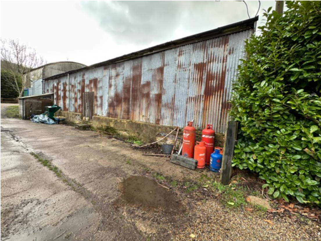
Photograph 7: Eastern aspect of the agricultural building, looking south
