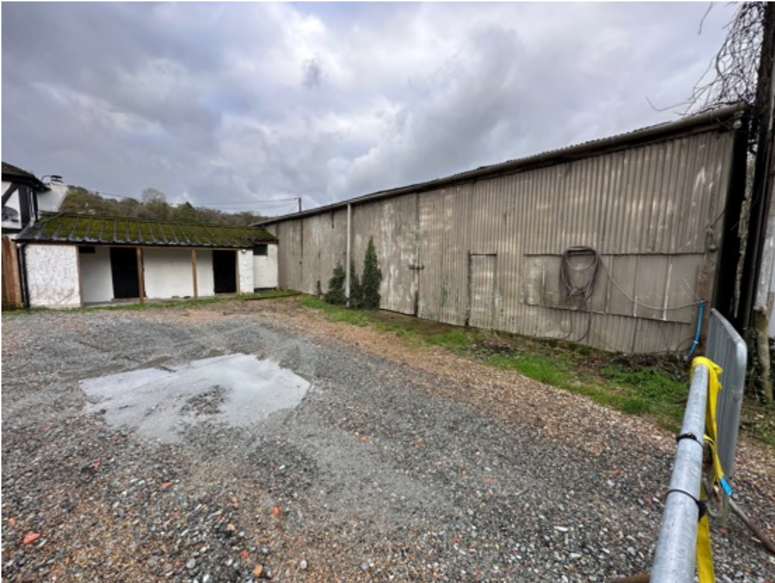
Photograph 5: Southern aspect of the stables and western aspect of the agricultural building
