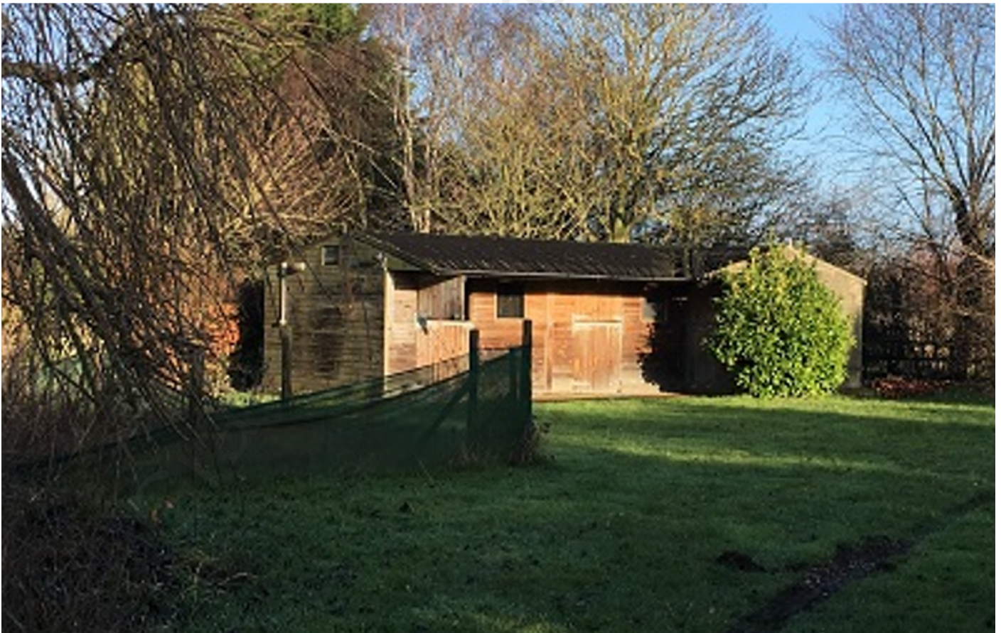
The stable building prior to its current alteration was as shown in the photograph below taken on 11.12.2019.
