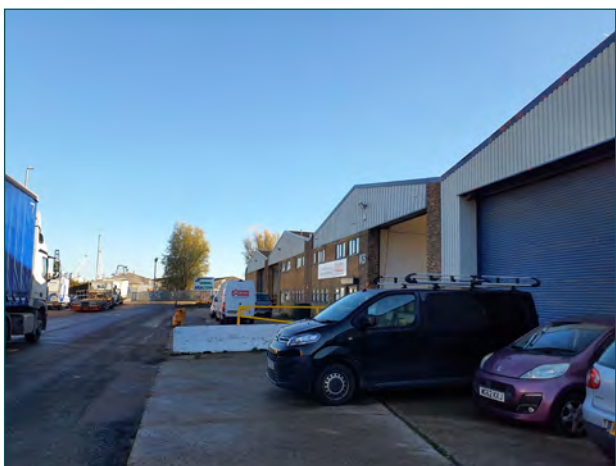
Photograph 3. Tarmac hardstanding located at the front of Building B1.
