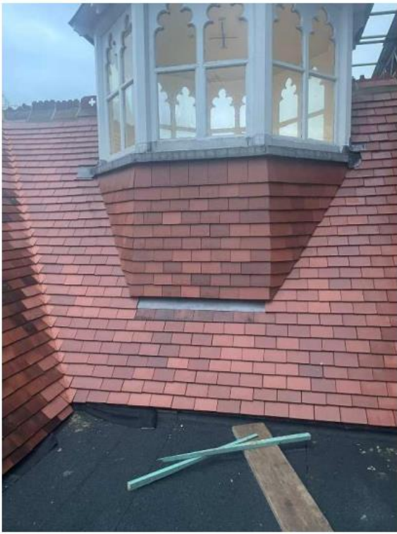
Previously Installed Tile – Image 1
