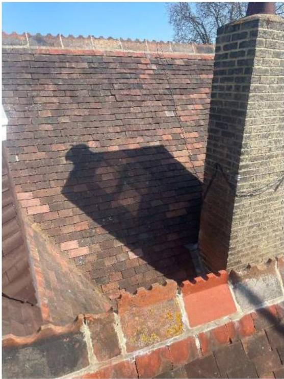
Newly Installed Tile – Image 2
