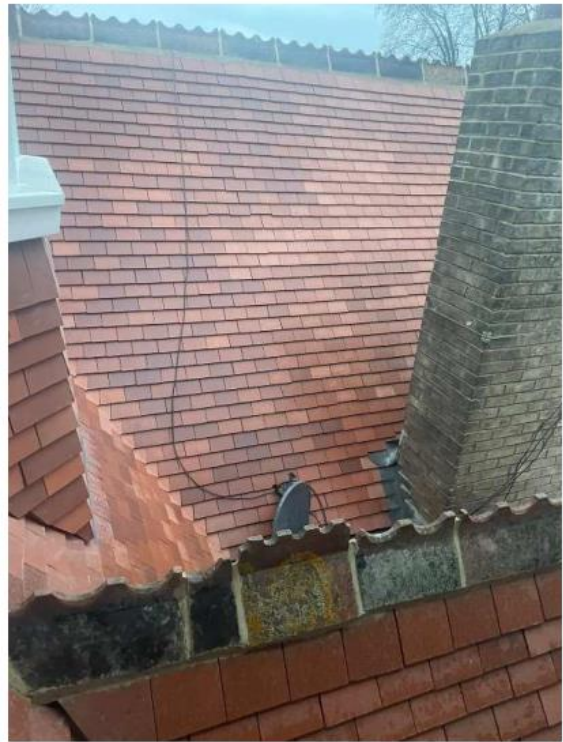
Previously Installed Tile – Image 2
