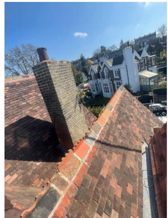
Newly Installed Tile – Image 4
