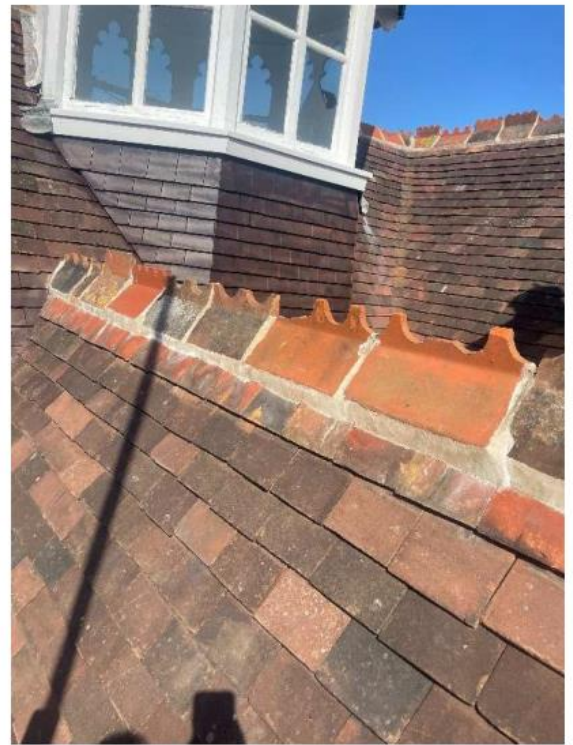
Newly Installed Tile – Image 3
