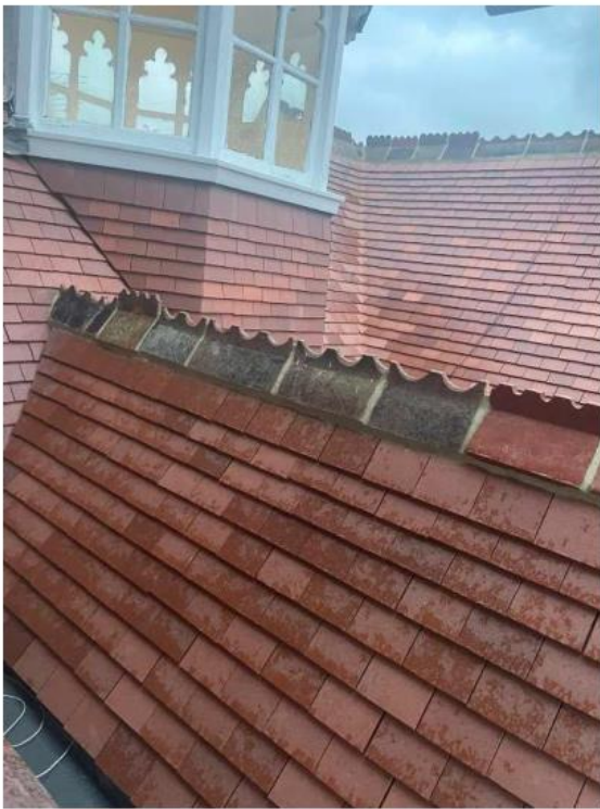
Previously Installed Tile – Image 3
