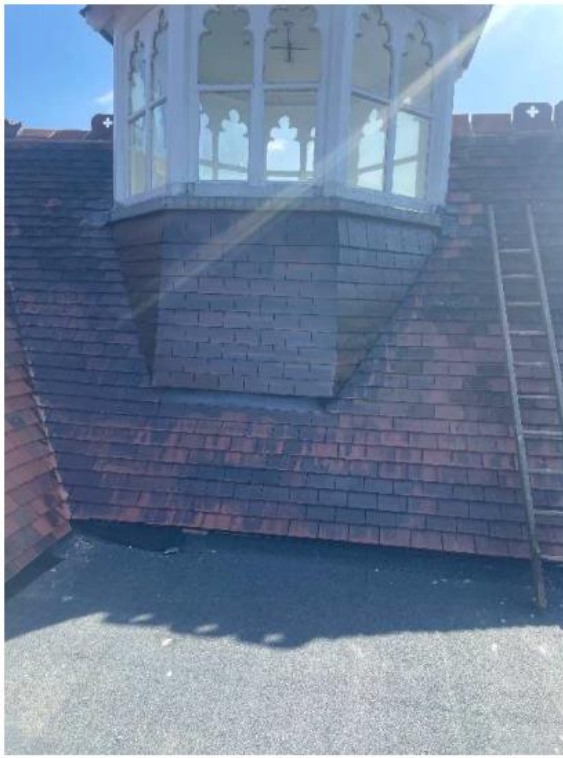
Newly Installed Tile – Image 1
