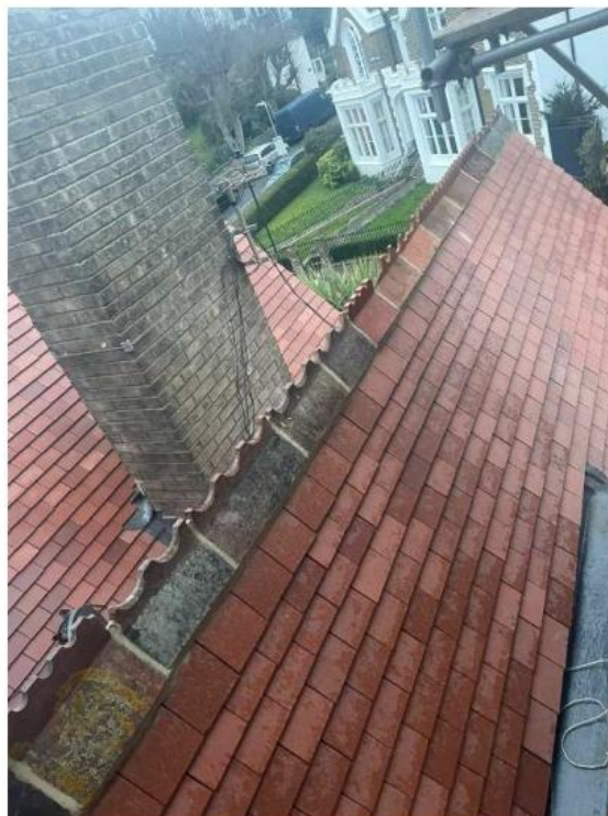
Previously Installed Tile – Image 4
