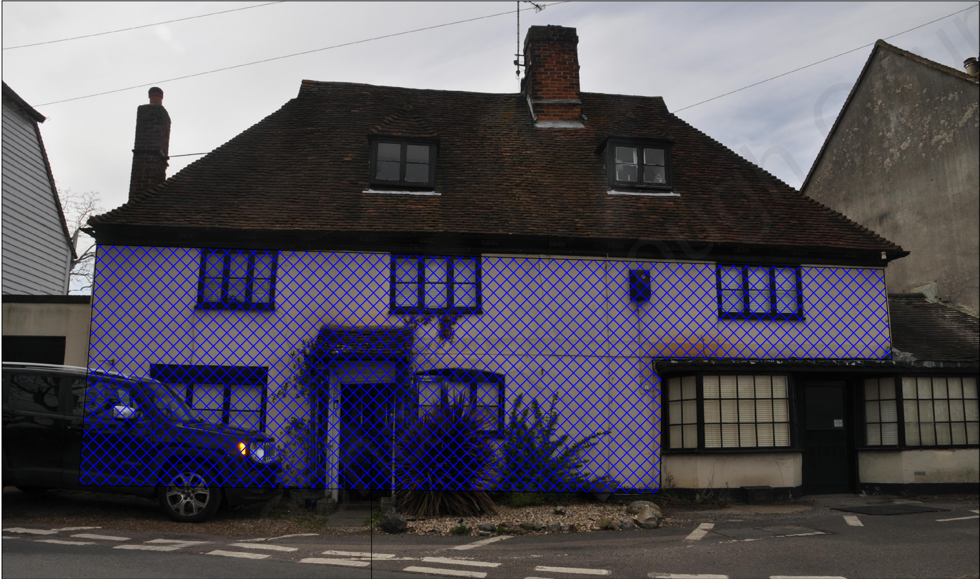
Area where render is proposed to be removed, repairs carried out and new lime render instated.
