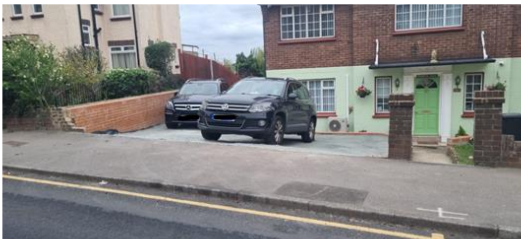
Source: Planning Enforcement, prior to rebuilding of dwarf front wall
