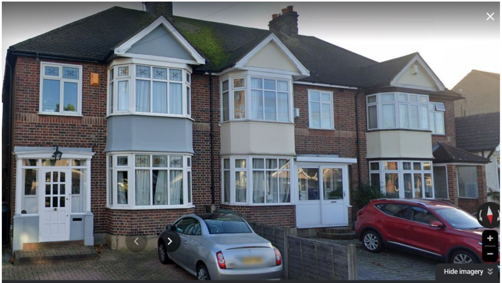
Document No. 1 – 14MA - Photo of Existing Property frontage including porch
