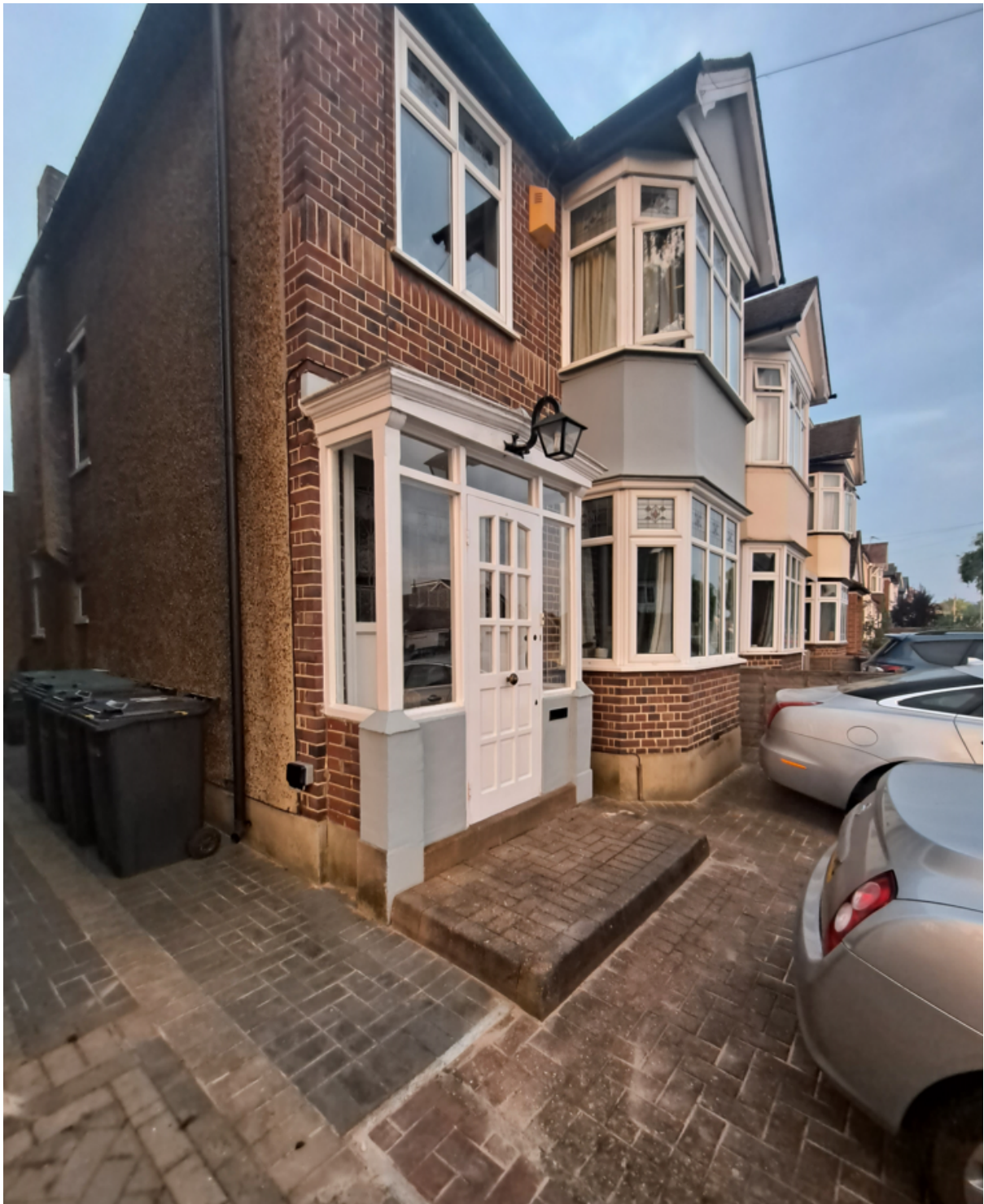
Document No. 2 – 14MA - Photo of Side elvation of Porch
