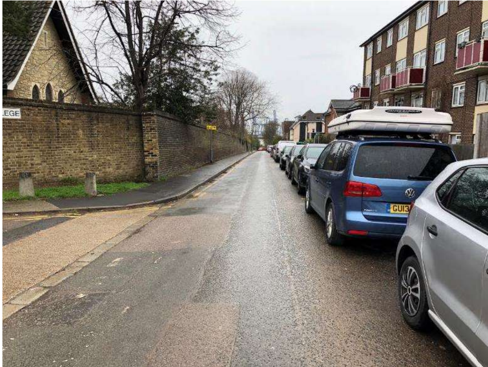
Figure 5-3 College Road Footway West side of Carriageway - Northbound View
