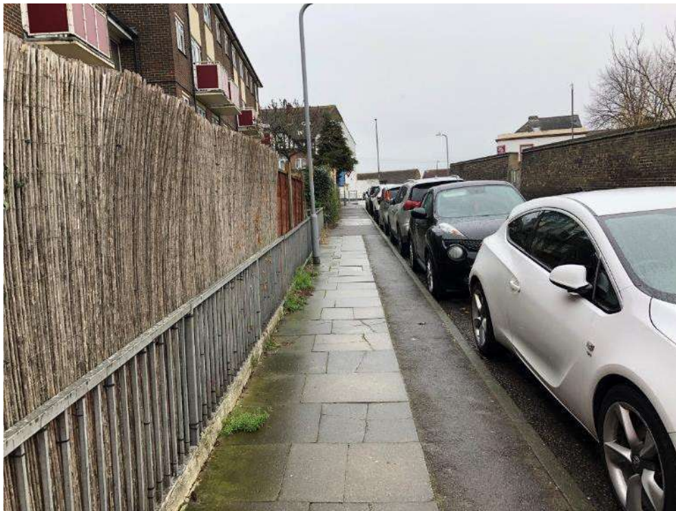
Figure 5-4 College Road Footway East side of Carriageway - Southbound View
