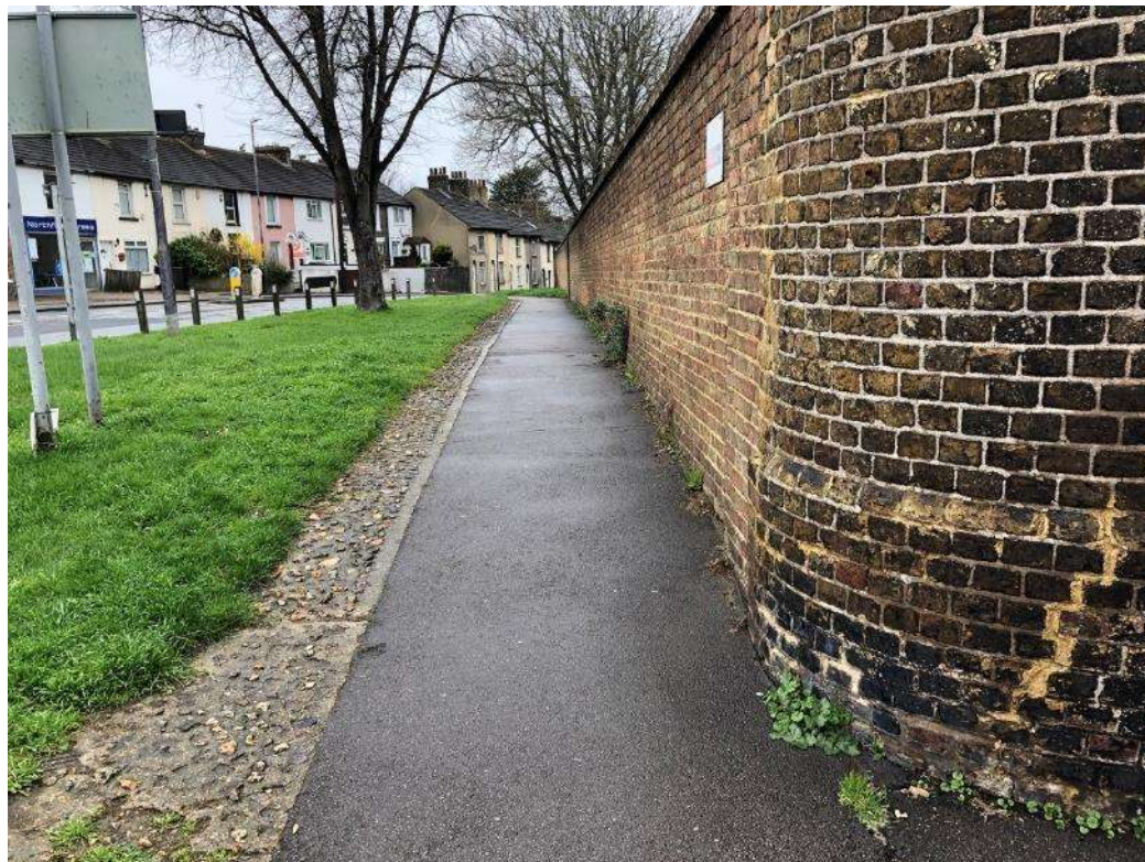
Figure 5-6 Stonebridge Road Footway
