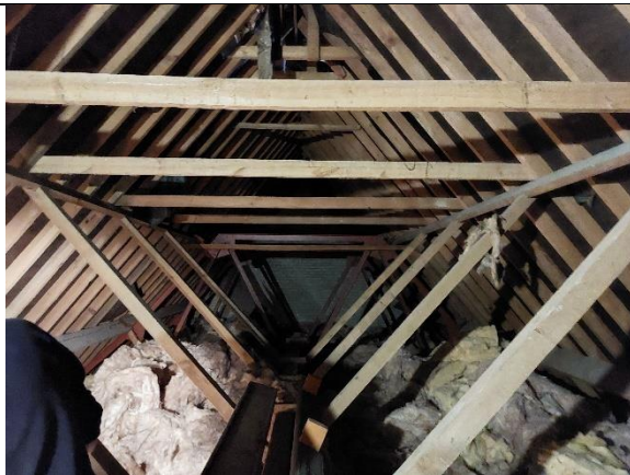
Image 13: internal roof space of the chapel.
