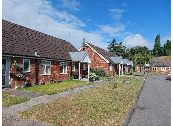
Image two: front of apartment blocks 3 – 7.
