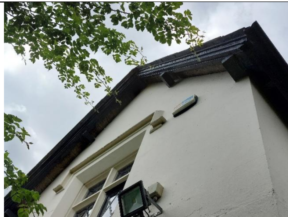
Image 14: the gable end of the Chaplain's house.
