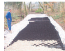
CellWeb during installation.
