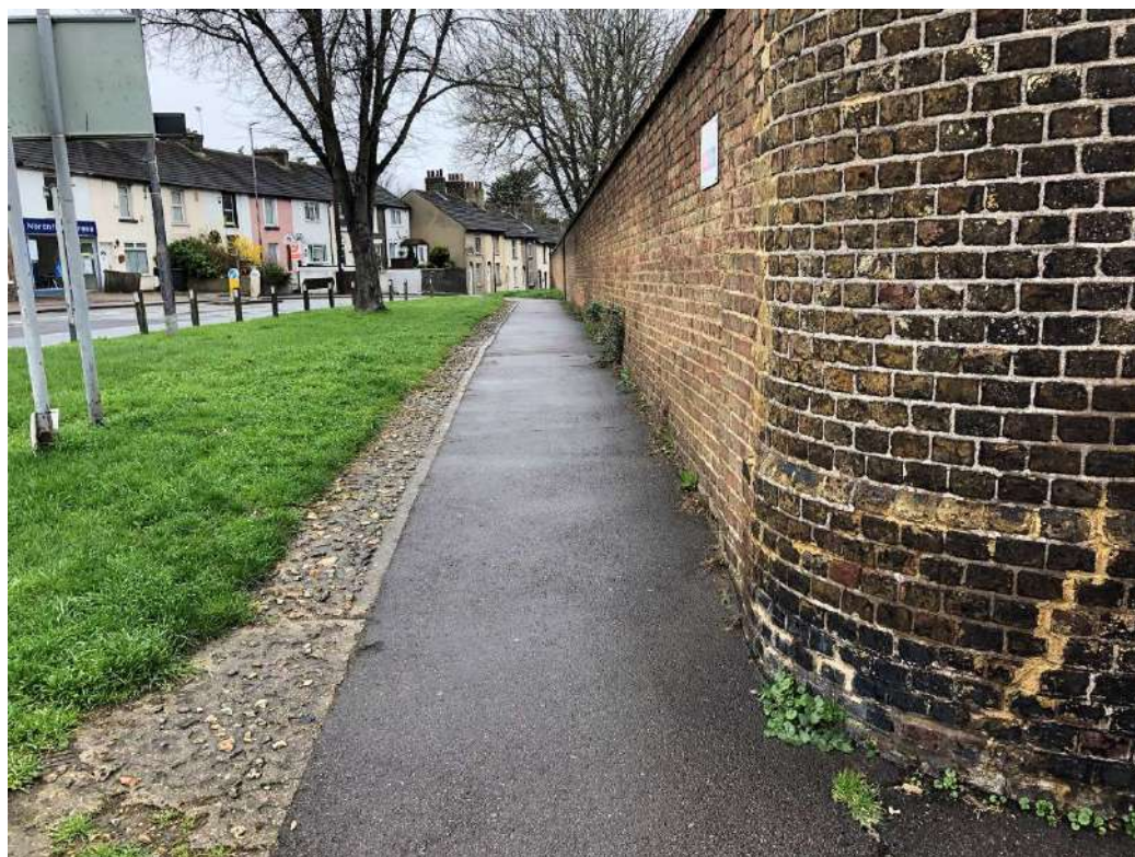
Figure 4-6 Stonebridge Road Westbound form College Road
