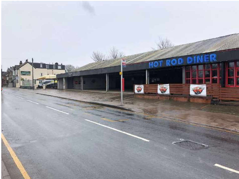
Figure 4-10 South Side of High Street East of the Site
