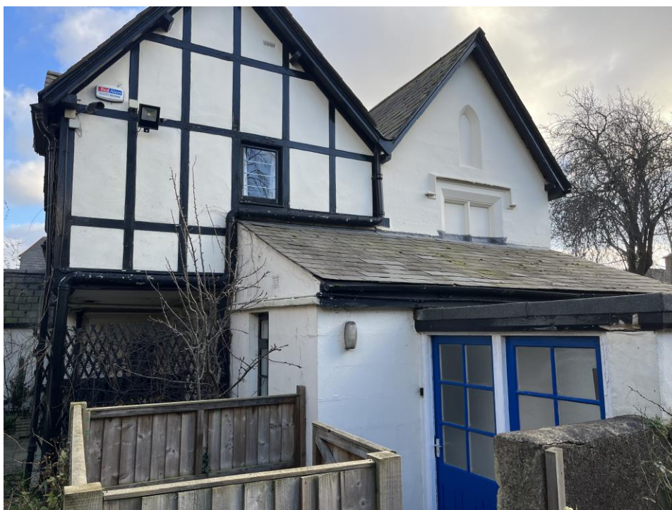
Plate 11: View looking SE towards the N-facing elevation of the Chaplain's House. Plate 12: View looking WSW across N-facing elevation of the Chaplain's House.
