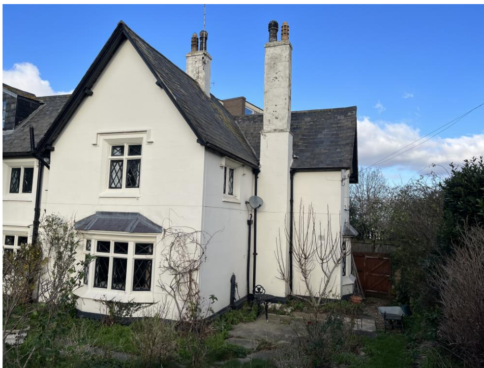
Plate 16: View looking NW towards the S-facing and E-facing elevations of the Chaplain's House.
