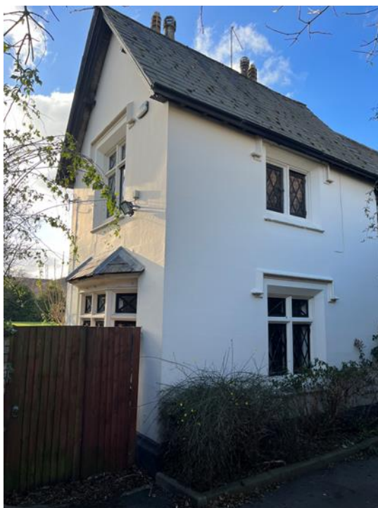
Plate 17: View looking SW towards the N-facing and E-facing elevations of the Chaplain's House
