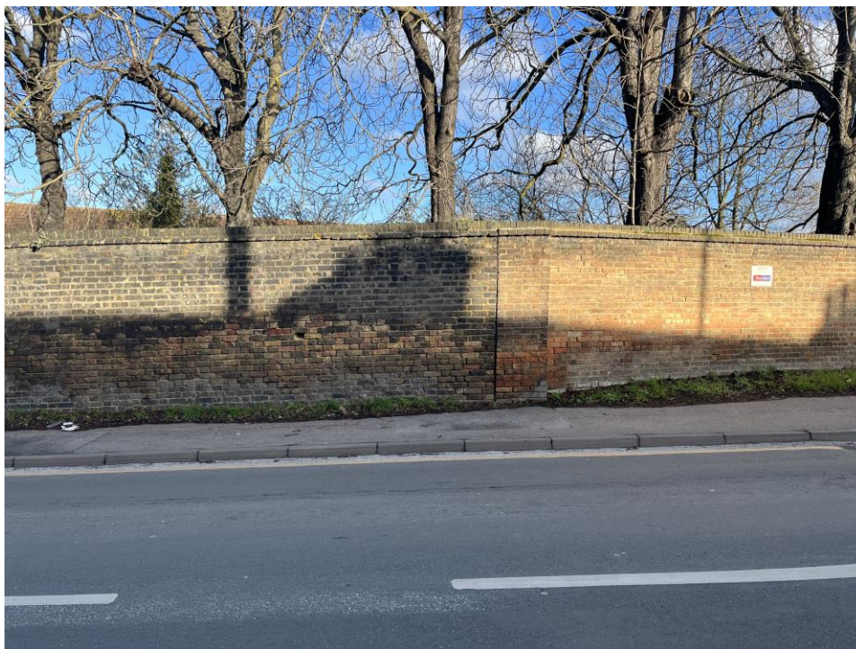
Plate 24: View looking N towards the boundary wall along Stonebridge Road.
