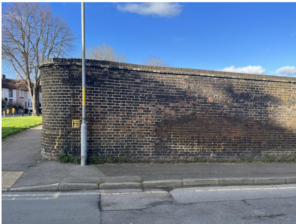
Plate 20: View looking W, towards the SE corner of the boundary wall.
