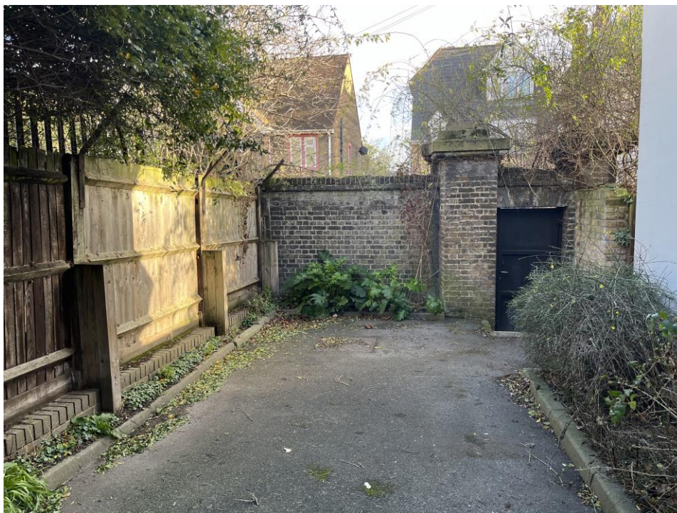
Plate 22: View looking E, towards the N end of the boundary wall along College Road.
