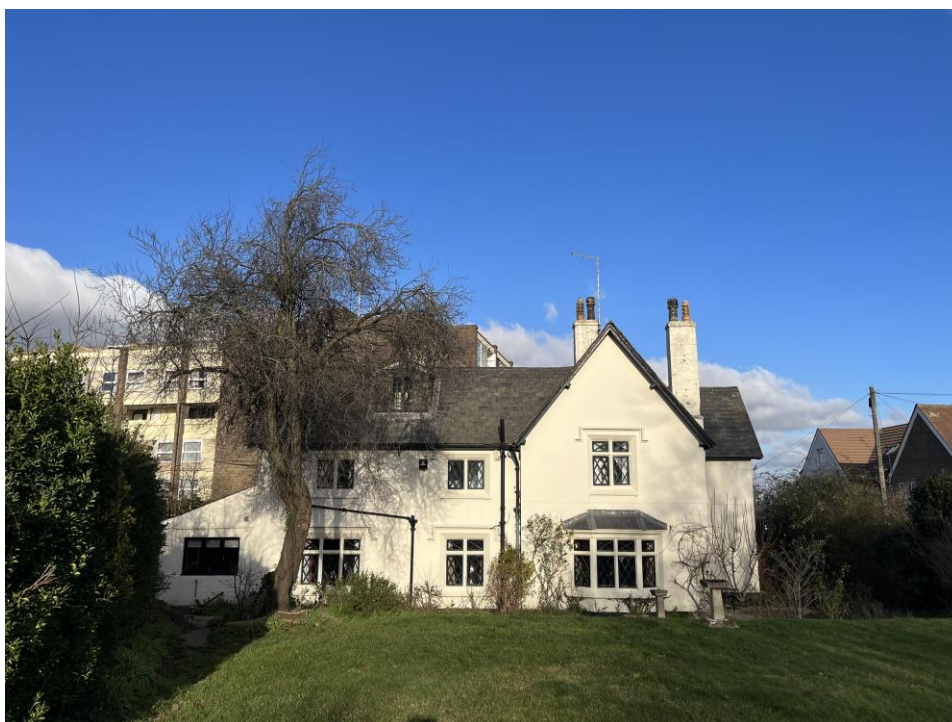
Plate 15: View looking N towards the S-facing elevation of the Chaplain's House.
