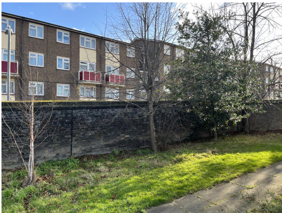
Plate 8: View looking SE parallel to College Road, showing the level of the ground in relation to the wall
