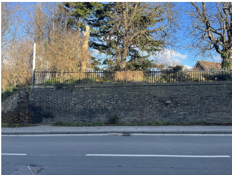
Plate 25: View looking N towards the boundary wall along Stonebridge Road.
