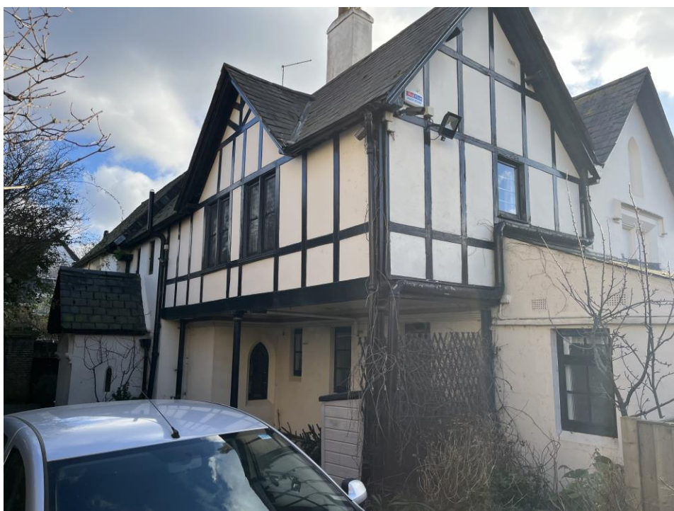
Plate 10: View looking ESE across the N-facing elevation of the Chaplain's House.
