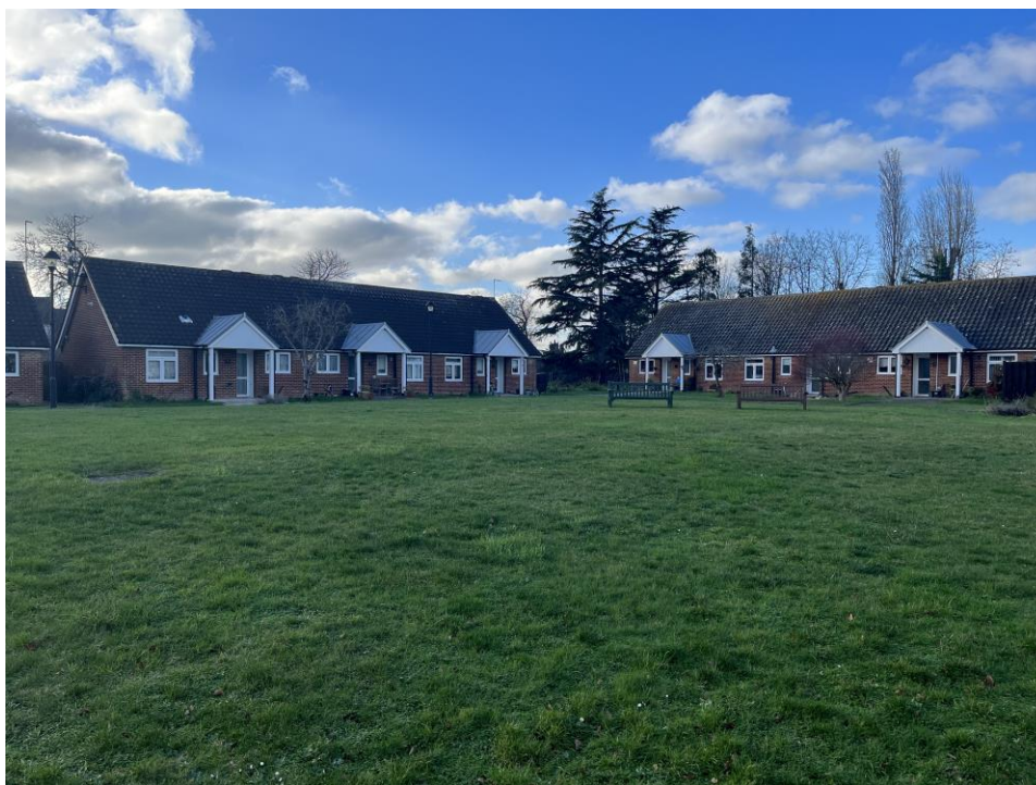
Plate 2: View looking SW across the central green.
