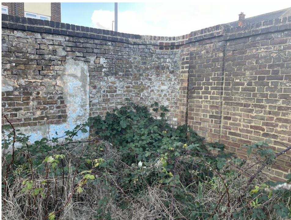
Plate 6: View looking SE, towards the SE corner of the boundary wall.
