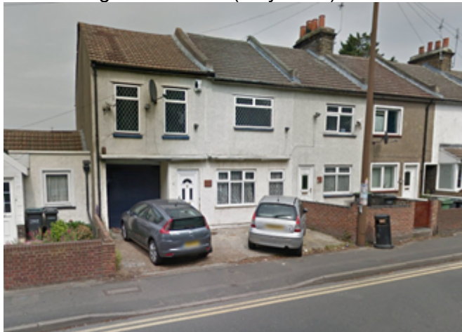
Pre-Existing Streetscene (May 2019)
