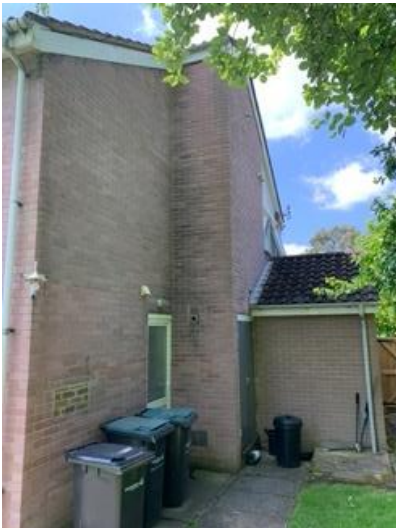
Photo 2.04 – Dunelm, Existing Side (facing Three Elms)
