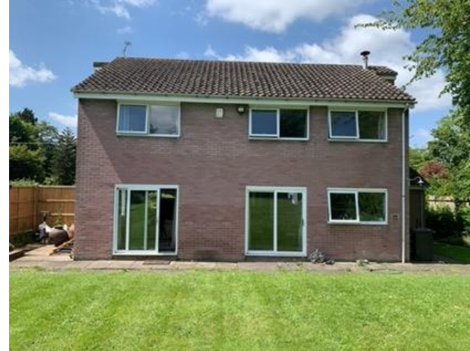
Photo 2.03 – Dunelm, Existing Rear
