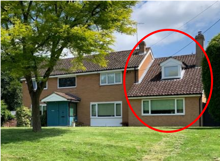
Photo 3.01 – Cedrus House (with side extension highlighted)
