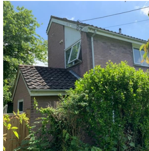
Photo 2.05 – Dunelm, Existing Side (facing Three Elms)
