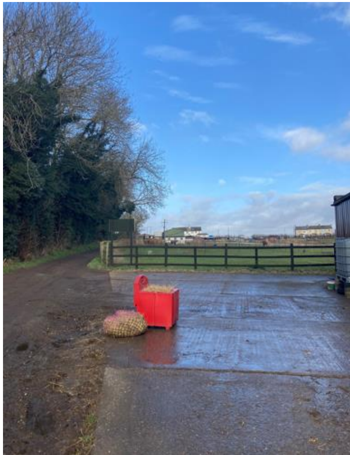
Front Forecourt Hardstand Area.
