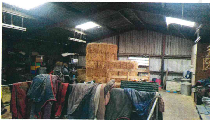
5. Internal above mezzanine level.
