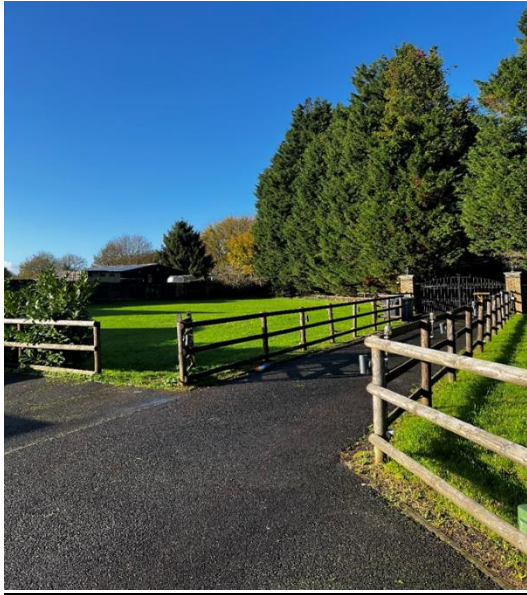
Driveway and entrance from main road
