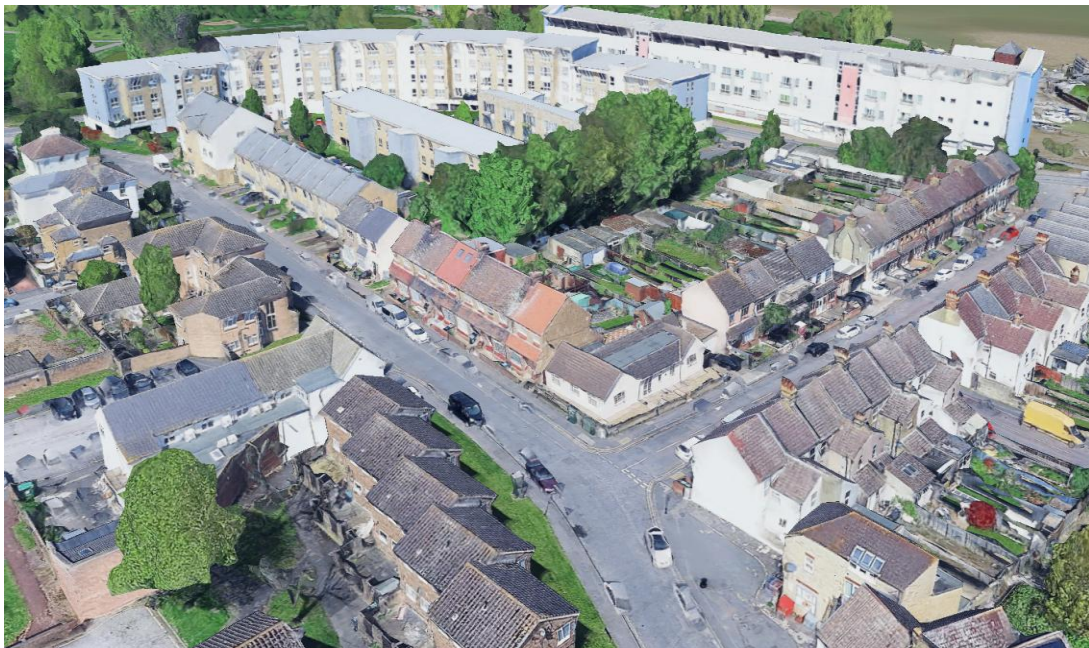
Image 2: Overhead view of site facing north west
