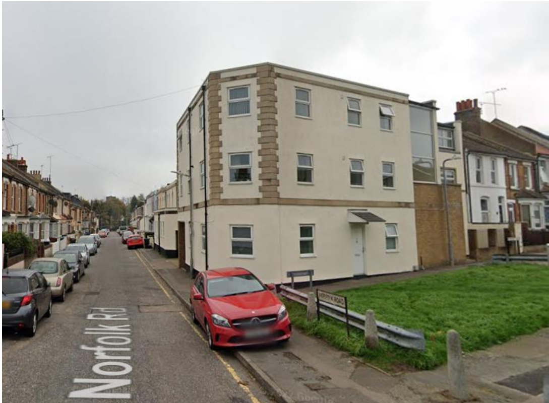
Image 11: Streetview image of the three storey Amber Court development from Albion Terrace/Norfolk Road.
