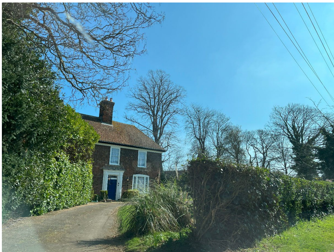
Figure 13: View of East Court Farmhouse, looking southeast
