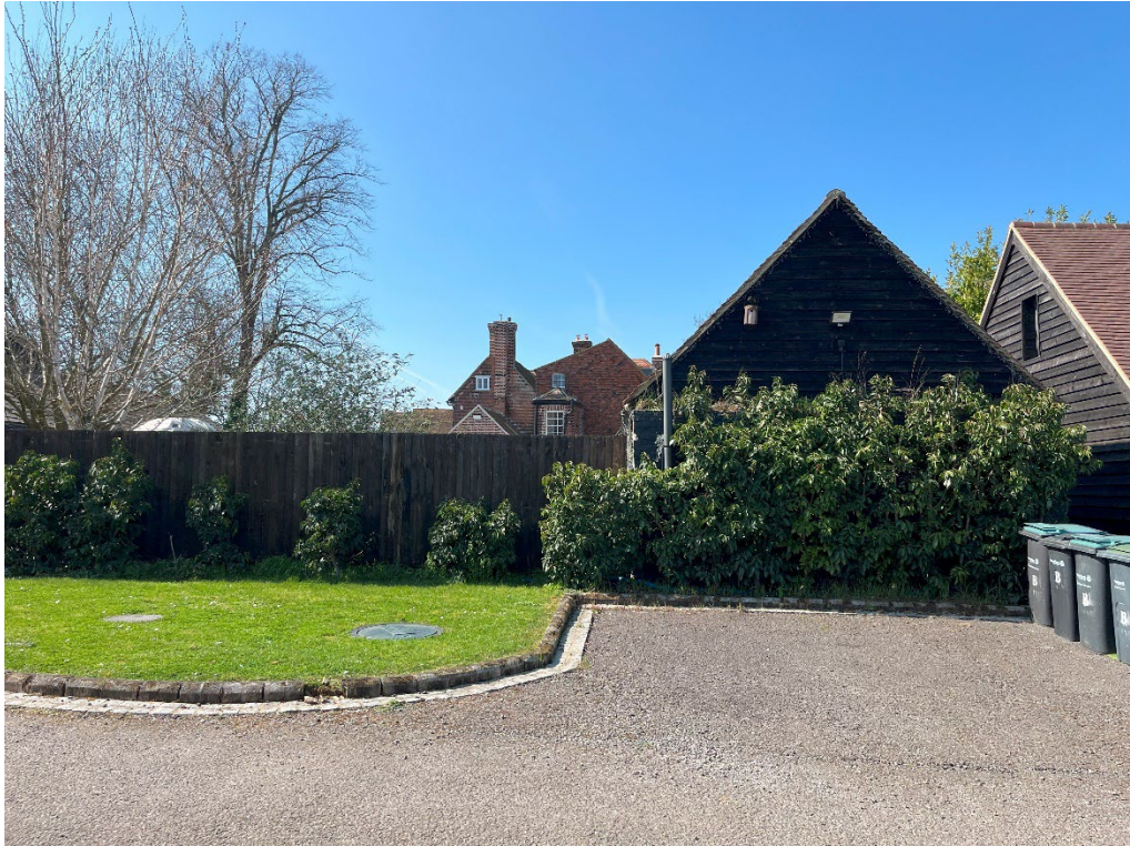
Figure 15: Rear, east, elevation of East Court Farmhouse and eastern gable end of historic farm building with fencing dividing off the land between the two parts of the farm.
