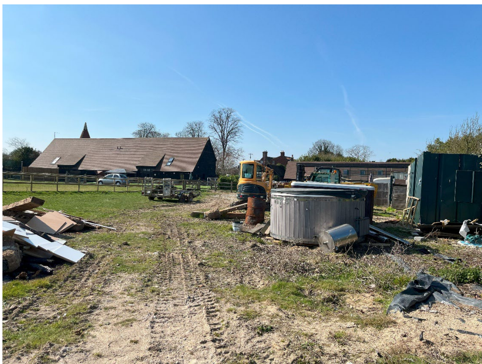
Photograph 8: View of the southern part of the Site, looking W
