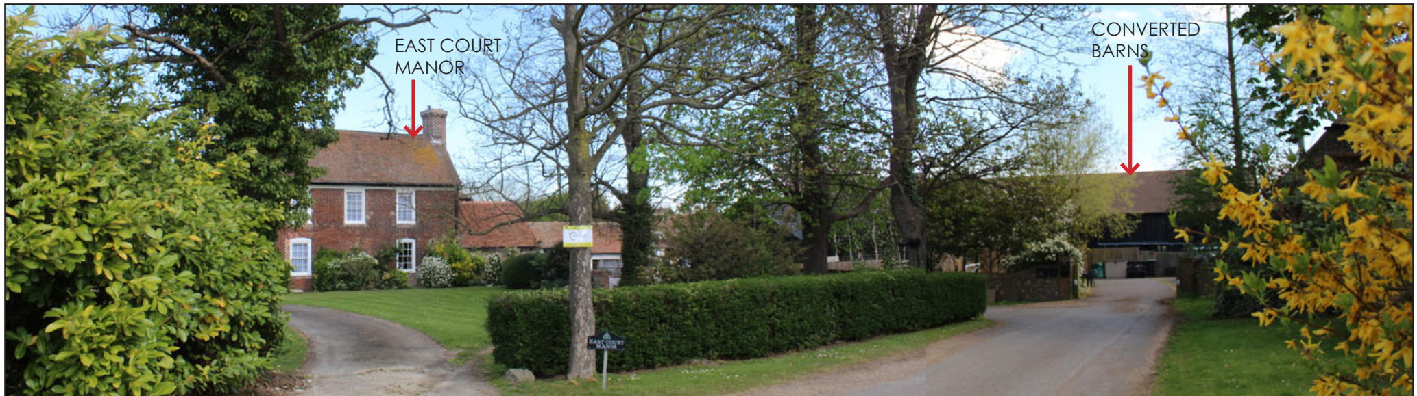
Photo 09. Taken from the access to East Court Manor, the house faces towards Church Lane, utilising what would have been the farm access to the now converted farm buildings. The well-vegetated gardens, orientation of the house and barns means that the proposals are not visible from this point.
