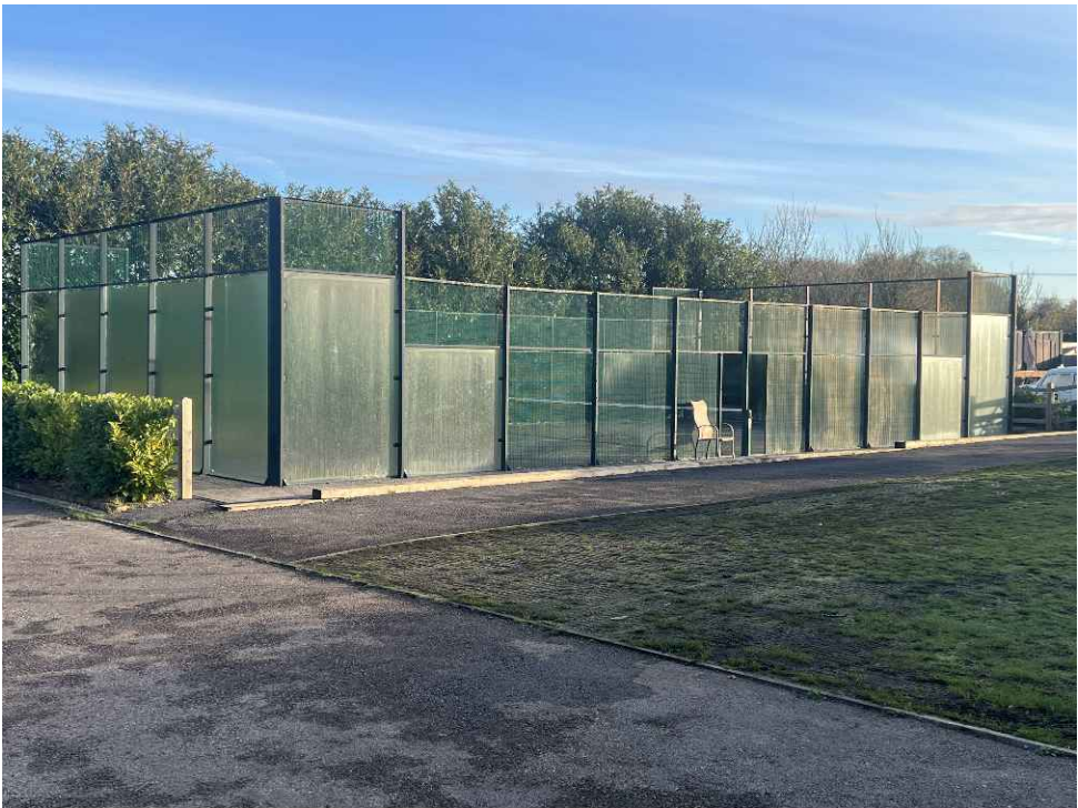
3. Existing tennis court to west of area for glamping pods.
