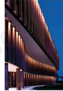
Light fittings to illuminate buildings mounted onto its facade (illuminated from top)
