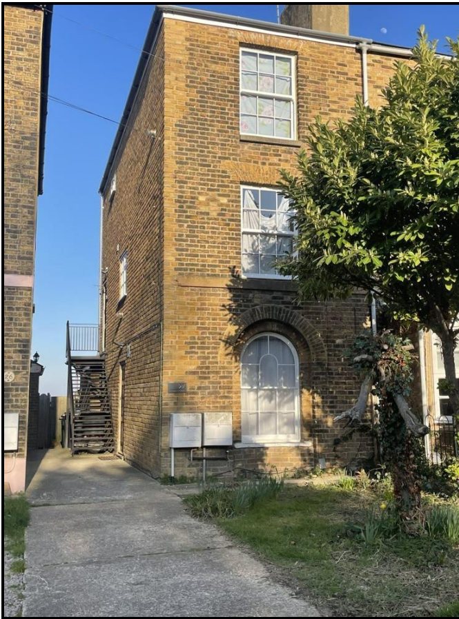
Image taken during a site visit on 13/03/23
