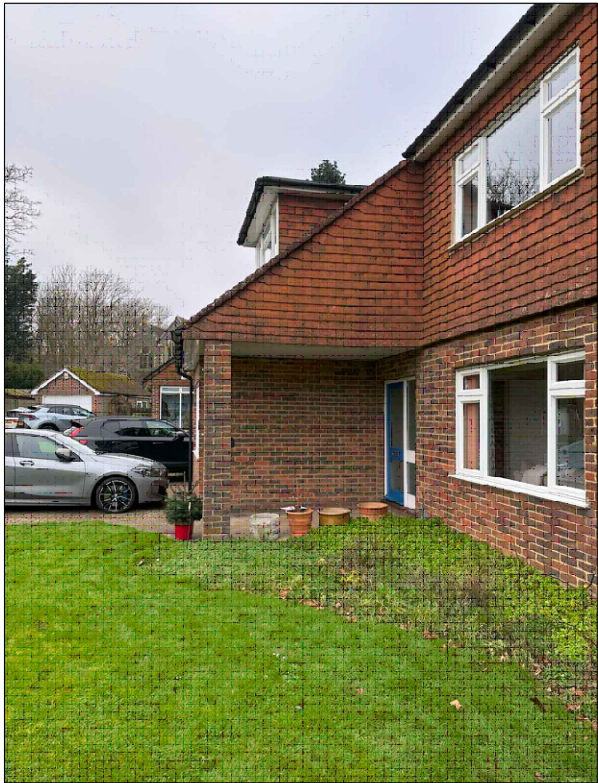
Existing Front Photograph
